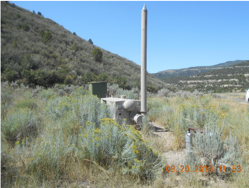
Flowline riser in lower right foreground.
