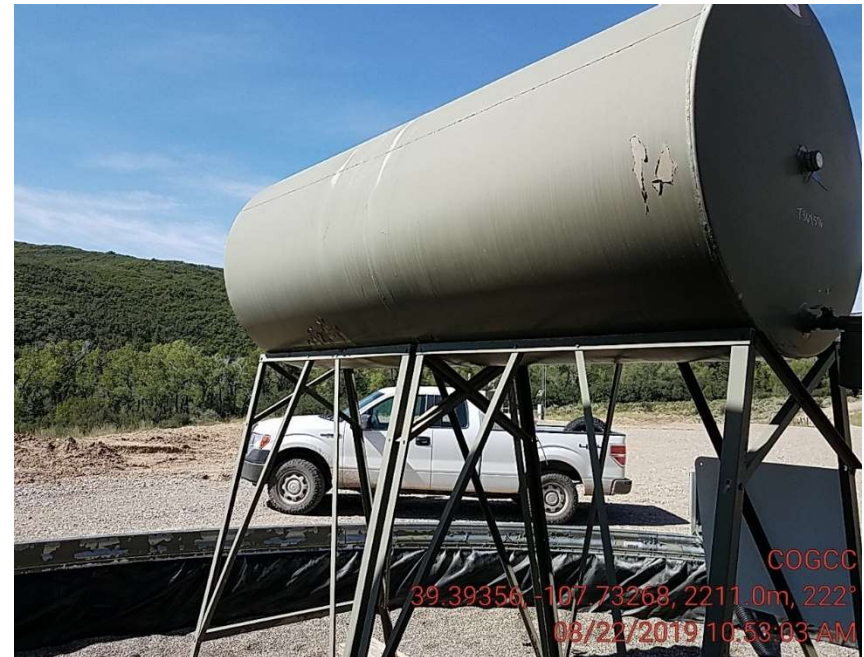
6 methanol tank missing labels
