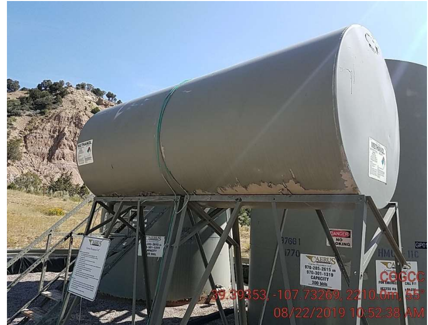
4 methanol tank missing labels
