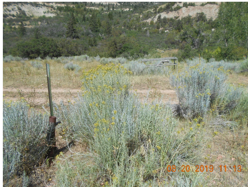
Anchor with marker. Flowline riser with pipe fence in background.
