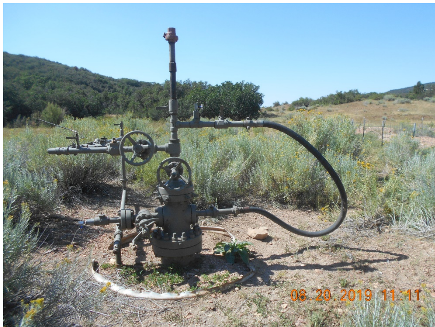
Wellhead (sign on tank)
