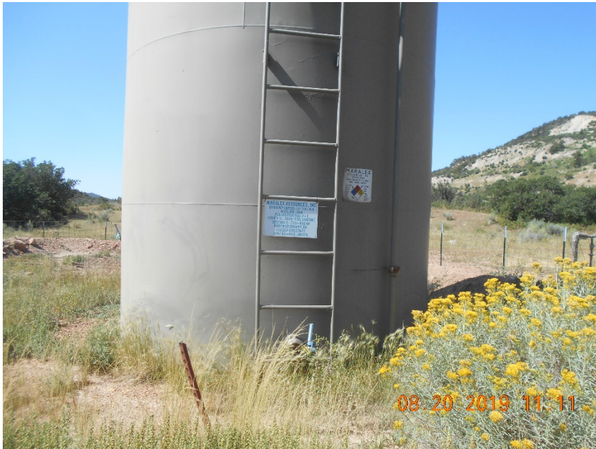
Tank battery with sign and labels
