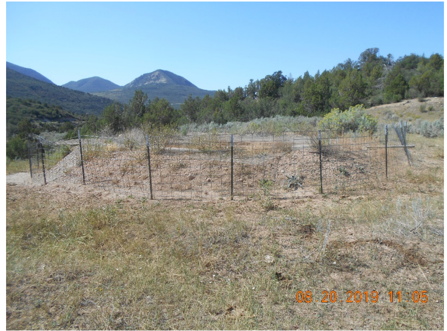
Blowdown pit with fence and netting.
