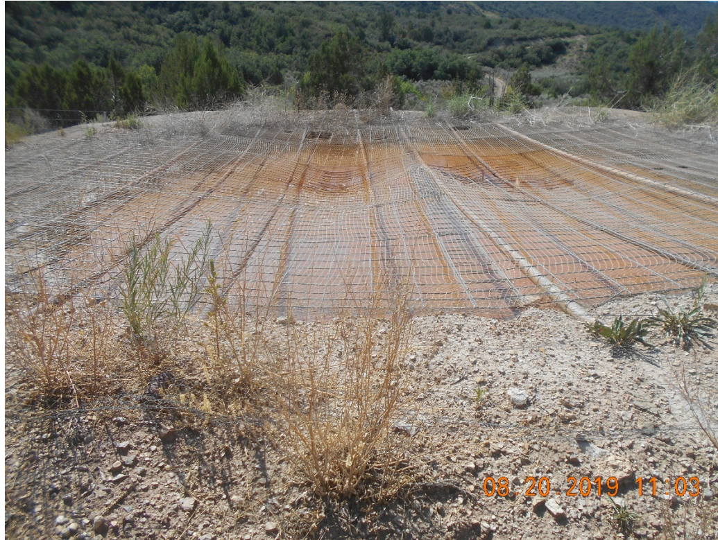
Blowdown pit with holes in netting.
