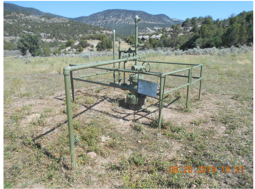
Wellhead with fence and sign
