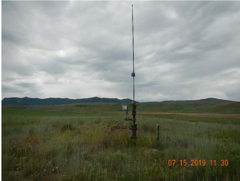
Photo 1. Unmarked riser at wellhead.
