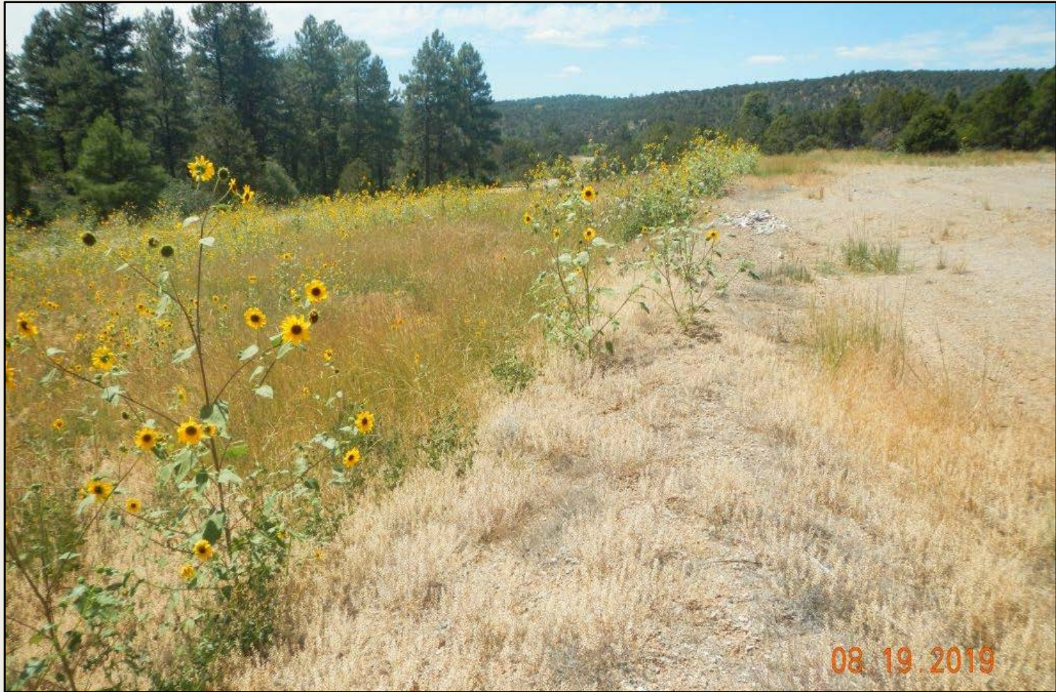
Photo 2. View of southern fill slope facing westward.
