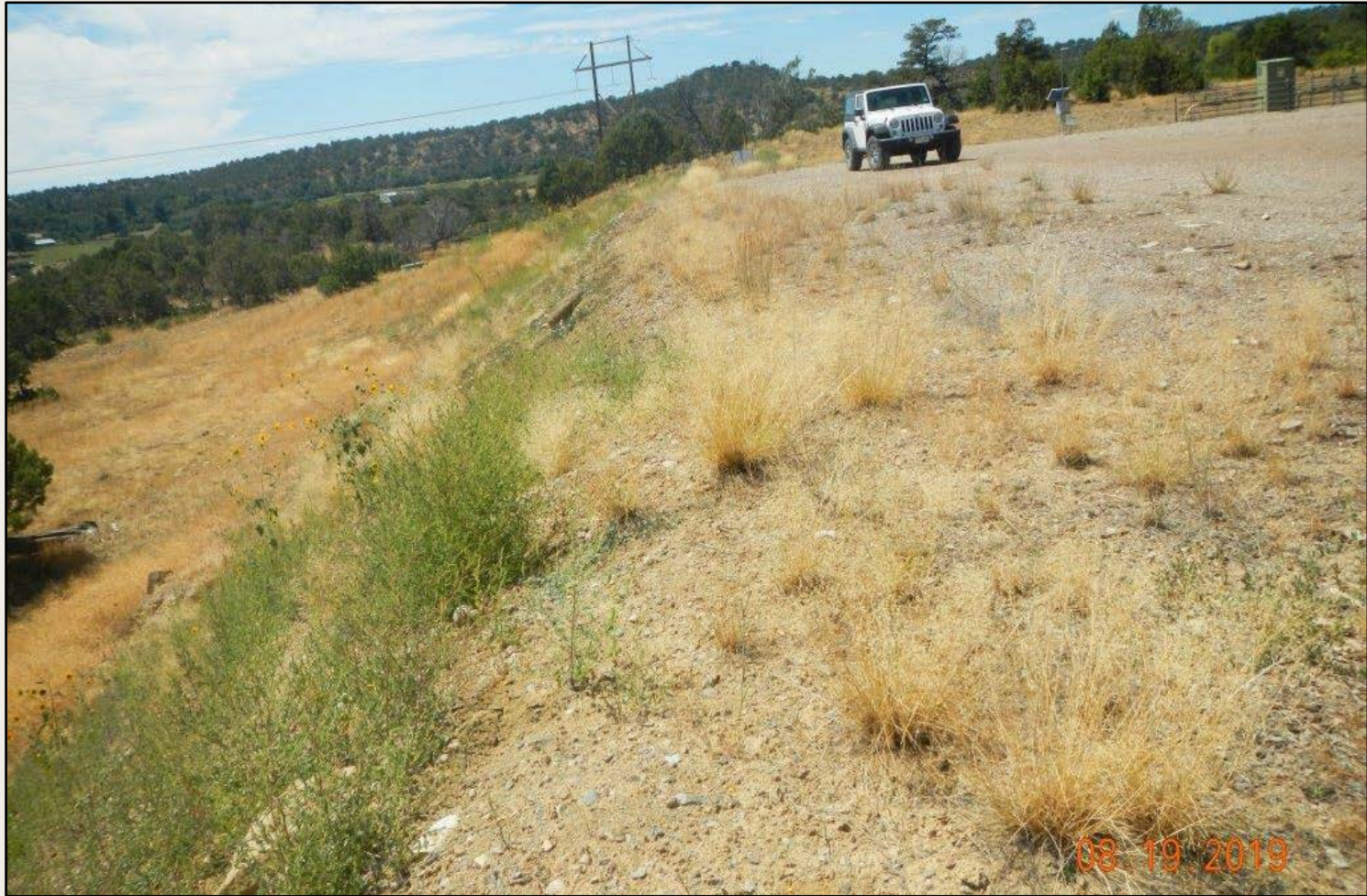
Photo 2. View of southern fill slope facing westward.
