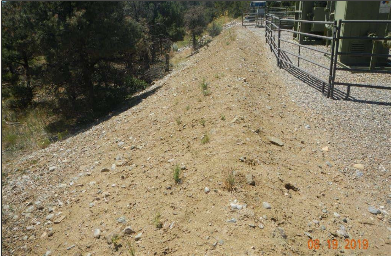
Photo 2. View of southern fill slope facing westward. Revegetation is sparse/young, but appears to be progressing. Some hydromulch remains on soil surface.
