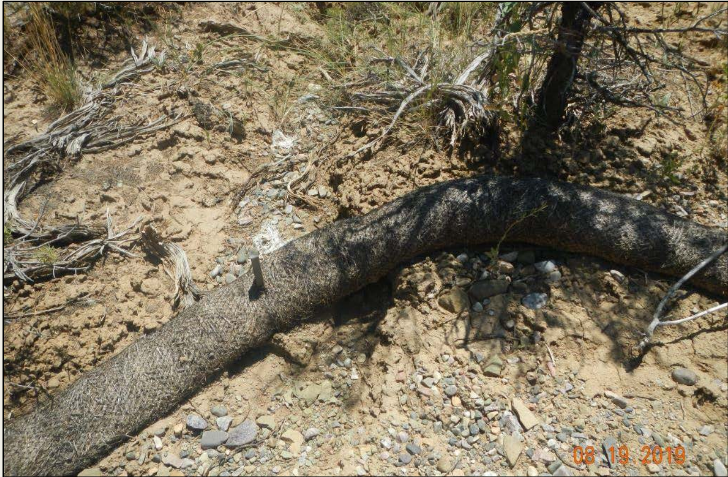
Photo 3. View of wattle in the southern project area that is no longer functioning. This is not an appropriate BMP for this area.
