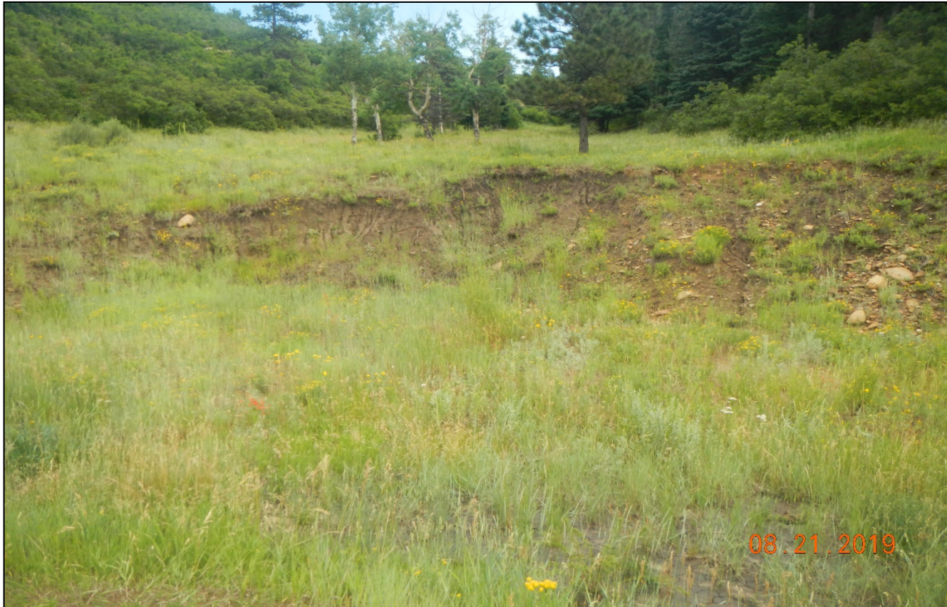
Photo 6. There is erosion along the cutslope at the north side of the location near the shallow pit.
