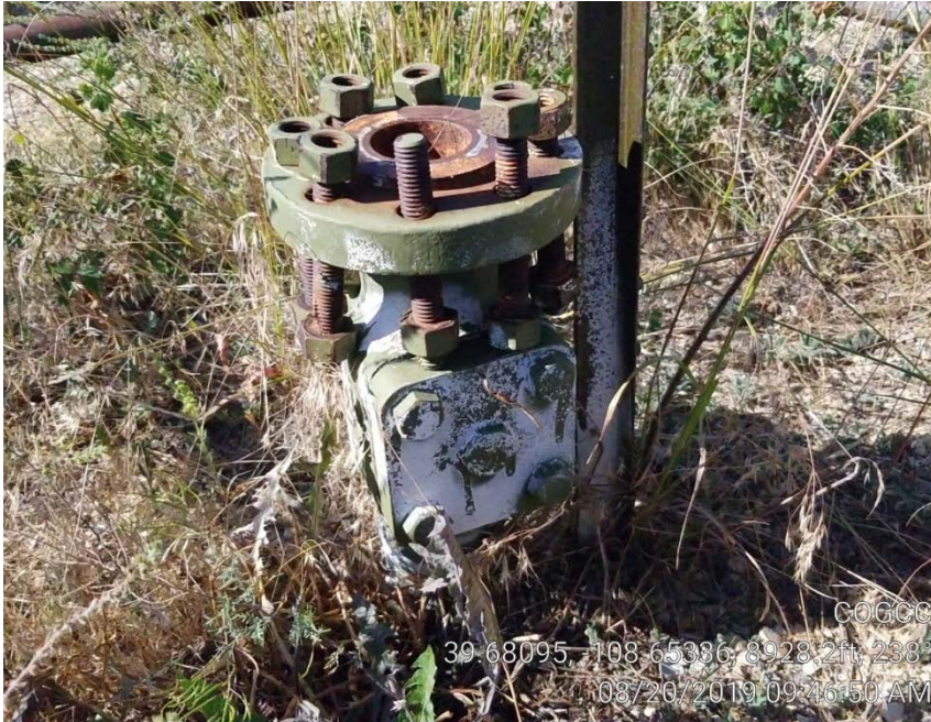
Photo 4. Flowline riser inside fenced area.
