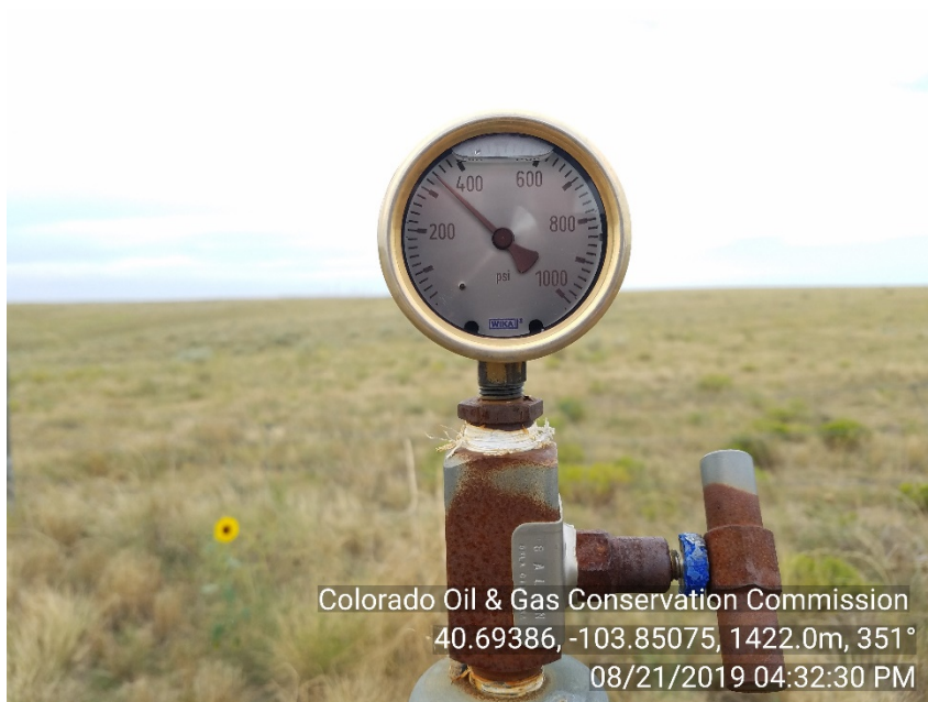
Photo #3 Lilli Unit 6-3 UIC - Injection Wellsite Temporarily Abandoned | TA Tbg. Press: 340#
