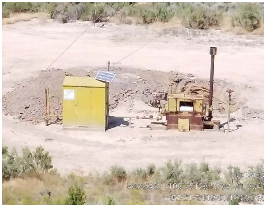
Photo 2. Separator, gas meter building, and pit.
