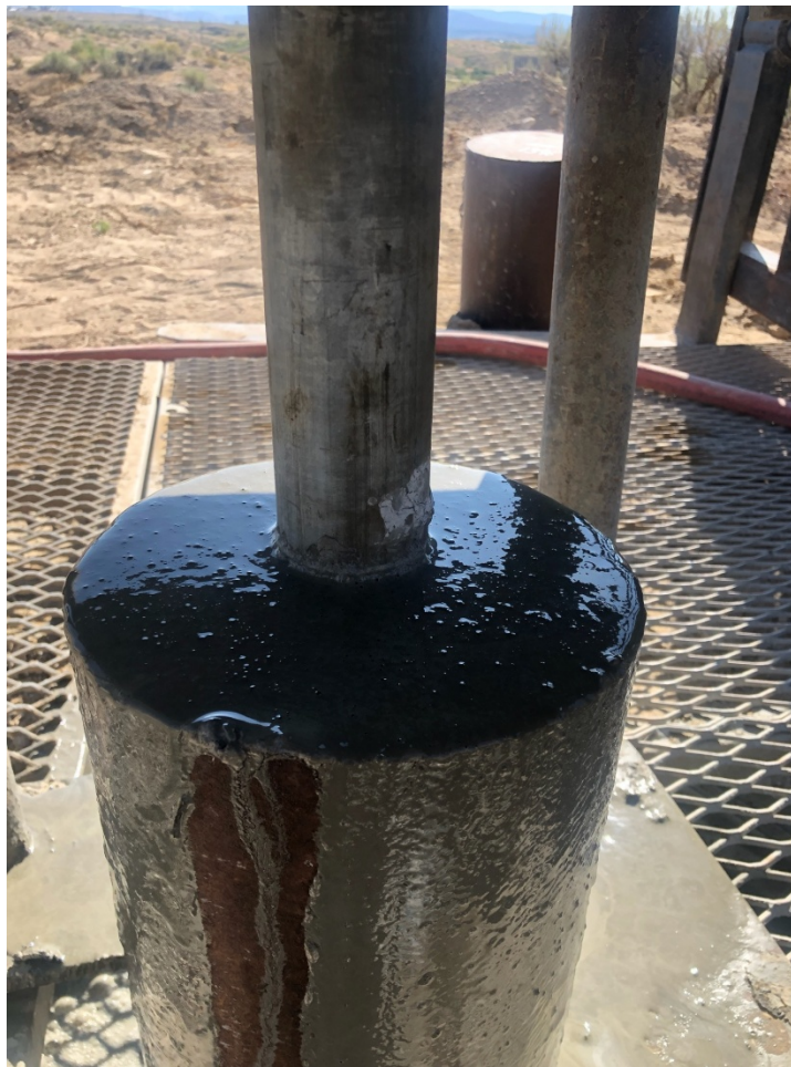
Photo 2. Well head with cement to surface & cement string not removed yet.
