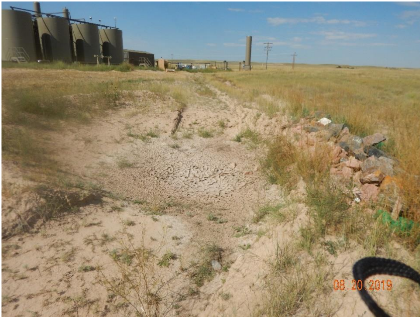
Photo 33: Photo of sediment trap on the north end of the location. See comments under photo 7. Photo also shows that the outlet of the sediment trap has been constructed at the same elevation as the adjacent ditches and berms, and will not allow for stormwater discharge.
