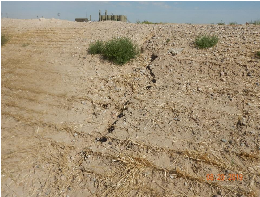
Photo 11: Photo taken from the south end of the pad. Photo shows erosion degradation on the slopes of the pad.
