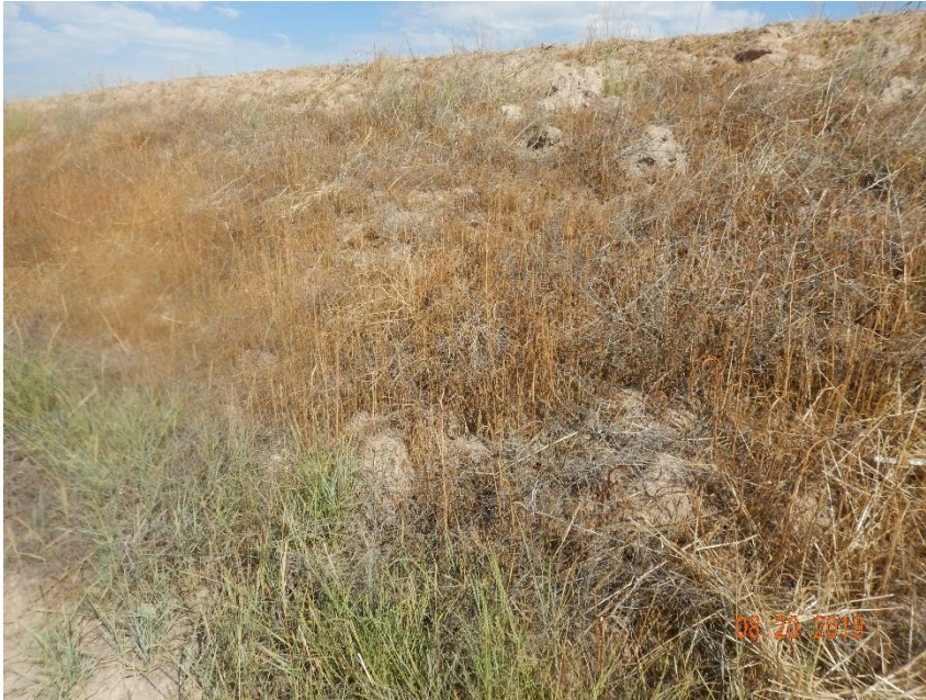
Photo 5: Photo taken from the south end of the topsoil stockpile. Weedy vegetative establishment on the topsoil stockpile. Photo also show no BMPs have been installed on the south facing slopes of the stockpile in accordance with 1002.c
