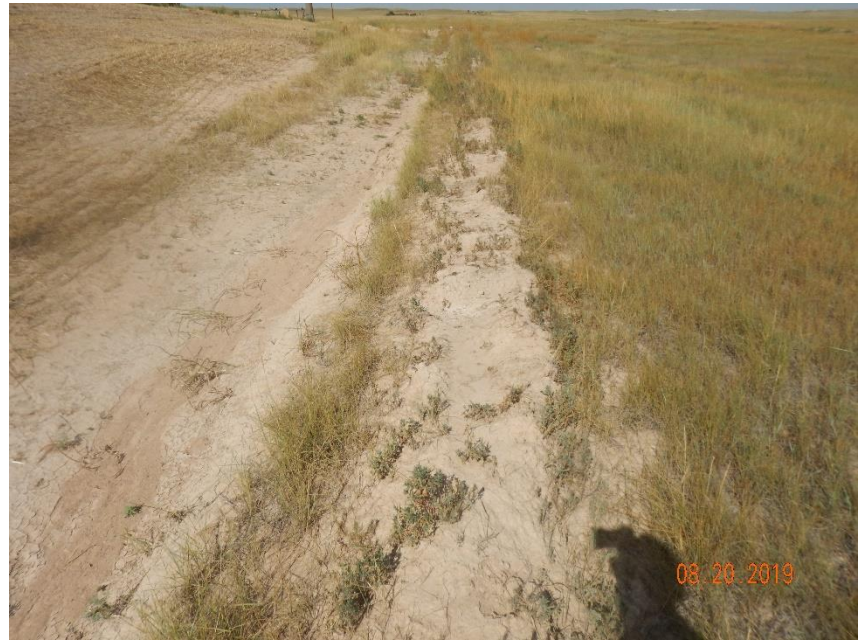
Photo 32: Photo shows perimeter stormwater ditch on the north end of the location. Photo shows stormwater ditch has not been constructed in accordance with good engineering practices, and has not been properly compacted/consolidated/stabilized. Photo also shows sediment due to stormwater erosion has filled the ditch.
