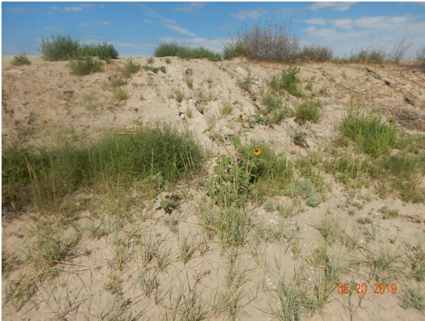
Photo 23: Photo taken from the east end of the pad, facing east. Photo shows erosion degradation on the slopes of the pad.
