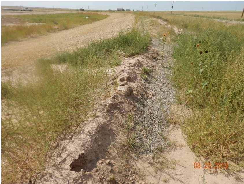
Photo 39: Photo shows perimeter stormwater ditch on the west end of the location. Photo shows stormwater ditch has not been constructed in accordance with good engineering practices, and has not been properly compacted/consolidated/stabilized. Photo also shows sediment due to stormwater erosion has filled the ditch.
