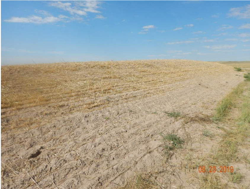
Photo 13: Photo taken from the north side of the soil stockpile. Photo shows Operator appears to be implementing BMPs to prevent weed establishment and to protect the stockpiled soils on the top, and northern facing slopes of the topsoil stockpile.
