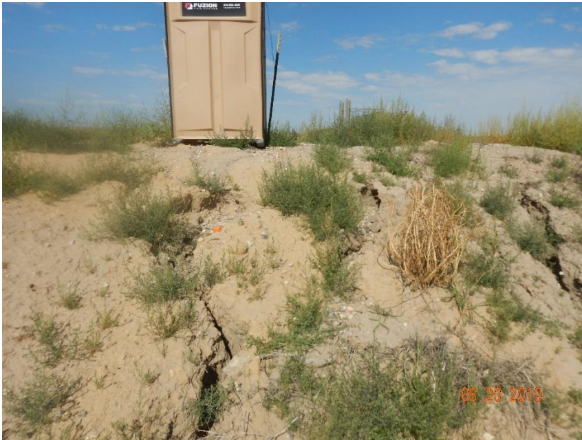
Photo 25: Photo taken from the east end of the location, facing west. Photo shows erosion degradation on slopes is beginning to cut under the porta-john on the east end of the location. Erosion degradation is compromising the stabilization of the porta-john and may result in tipping and spilling contents.
