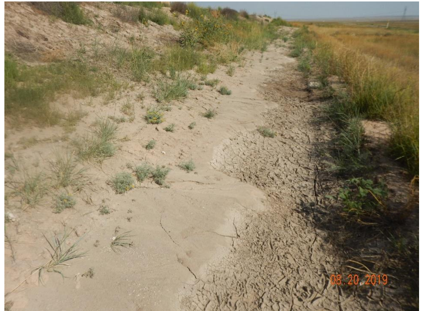
Photo 24: Photo shows sediment deposition has filled the stormwater ditch.
