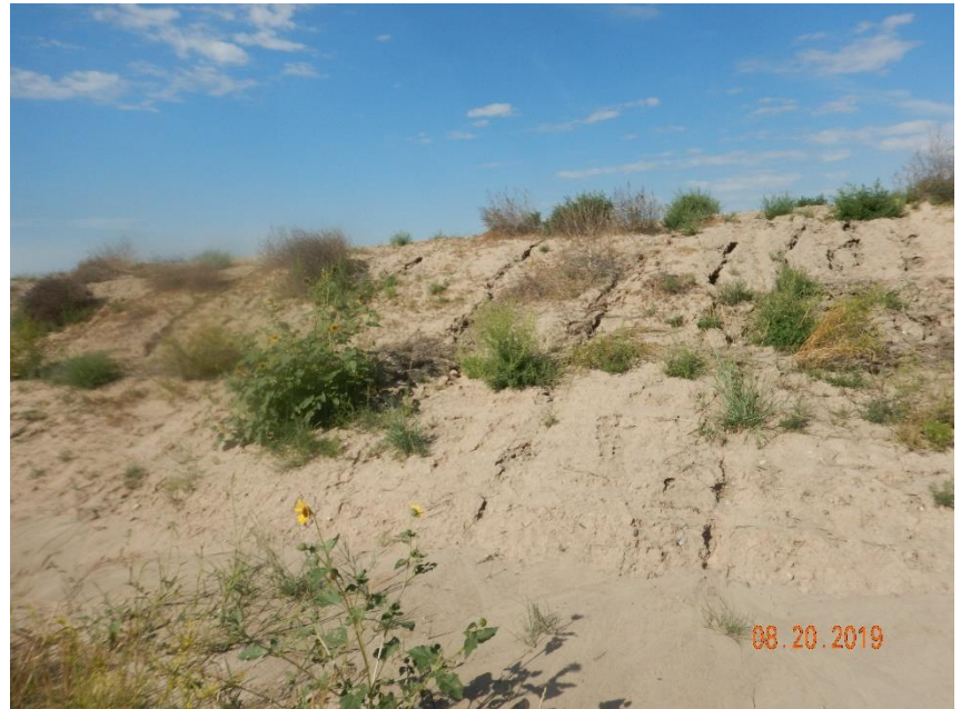
Photo 18: Photo taken from the east end of the pad, facing west. Photo shows erosion degradation on the slopes of the pad.
