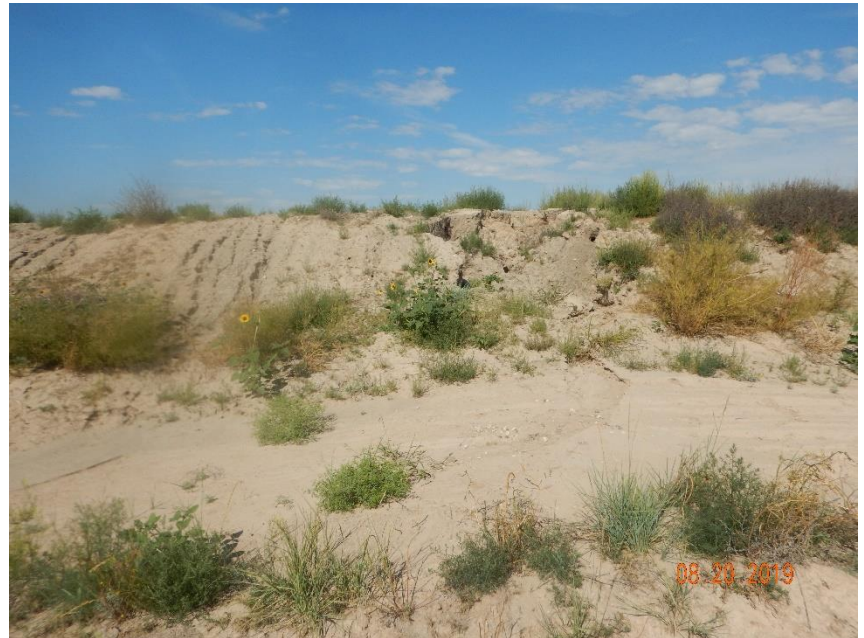
Photo 16: Photo taken from the east end of the pad, facing west. Photo shows erosion degradation on the slopes of the pad.
