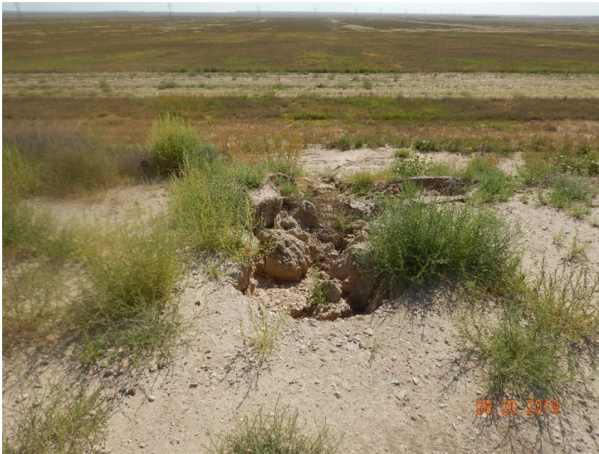
Photo 19: Photo taken from the east end of the pad, facing east. Photo shows erosion degradation on the slopes of the pad.
