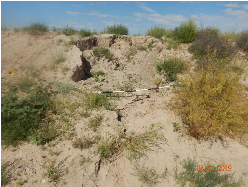
Photo 21: Continued from photo 20. Photo shows erosion degradation on the slopes of the pad. Two (2) meter Robel-pole in photo used for reference.
