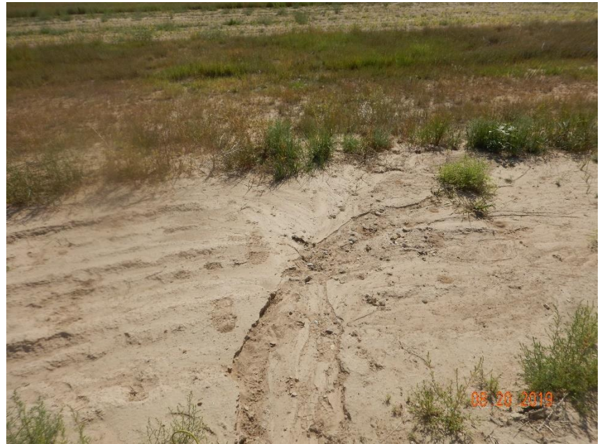
Photo 22: Continued from photo 21. Photo shows sediment has filled ditch. Photo also shows sediment discharge off location.
