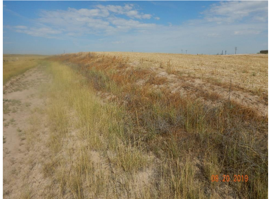
Photo 6: Continued from photo 5. Operator appears to be implementing BMPs to prevent weed establishment and to protect the stockpiled soils on the top, and northern facing slopes of the topsoil stockpile.
