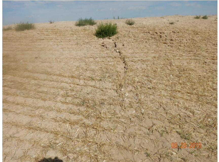
Photo 14: Photo taken from the south end of the pad. Photo shows erosion degradation on the slopes of the pad.
