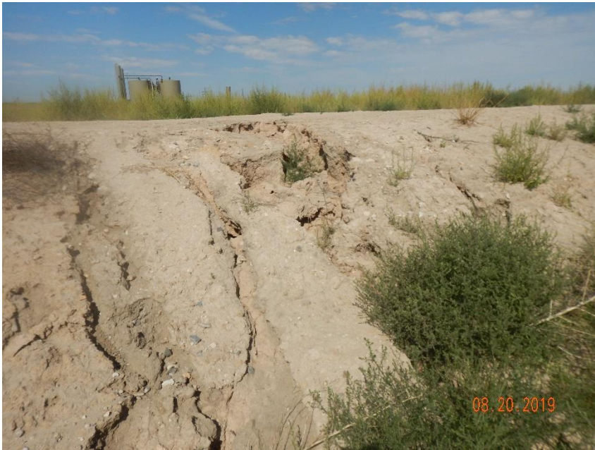
Photo 27: Photo taken from the east end of the pad, facing east. Photo shows erosion degradation on the slopes of the pad.
