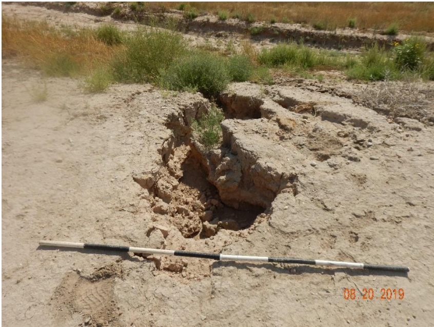
Photo 29: Photo taken from the east end of the pad, facing east. Photo shows erosion degradation on the slopes of the pad. Two (2) meter Robel-pole in photo used for reference.
