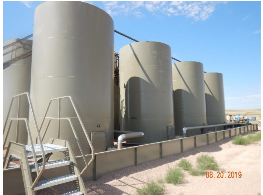
Photo 48: Photo taken from the tank battery. Photo shows tanks missing required labeling in accordance with 210.b
