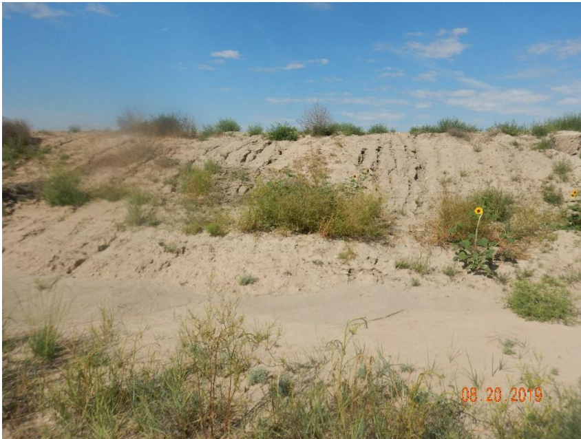
Photo 17: Photo taken from the east end of the pad, facing west. Photo shows erosion degradation on the slopes of the pad.
