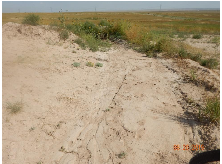
Photo 30: Photo taken from the northeast end of the location, facing north. Photo shows stormwater ditch has filled with sediment. Photo also shows sediment trap. See comments under photo 7 for comments regarding sediment traps on location.
