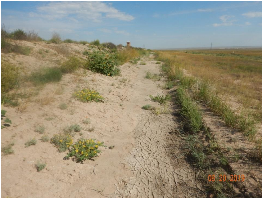
Photo 15: Photo taken from east end of the location, facing north. Photo shows stormwater ditch has not been constructed in accordance with good engineering practices, and has not been properly compacted/consolidated/stabilized. Photo also shows sediment due to stormwater erosion has filled the ditch.
