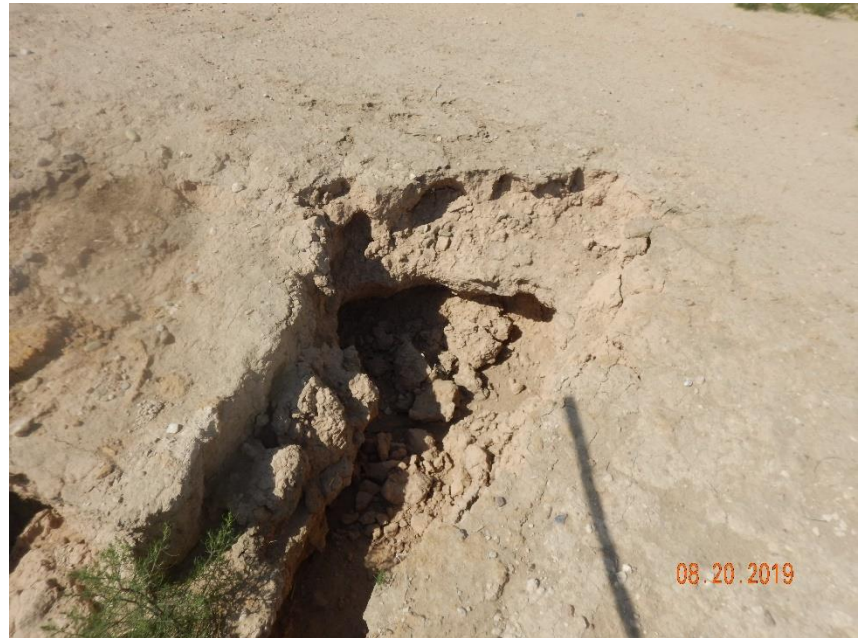
Photo 28: Photo taken from the east end of the pad. Photo shows erosion degradation on the slopes of the pad.
