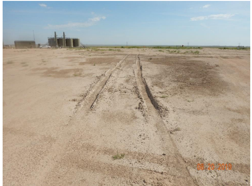
Photo 42: Photo taken from the southern are of the pad, facing northeast. Photo shows evidence of stormwater ponding on pad and vehicle tracking. Insufficient stormwater controls in place to allow for sediment laden free stormwater discharge from the location. BMPs need to be in place to 1) mitigate ponding, 2) prevent potential industrial pollutant contact and 3) to allow for sediment laden-free stormwater discharge from the location.
