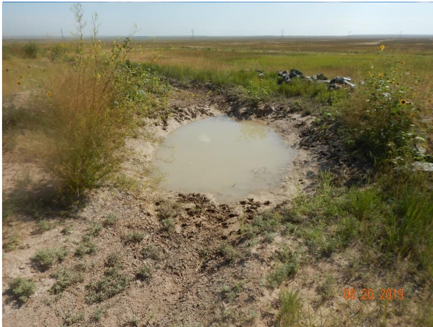
Photo 7: Photo taken from the sediment trap on the southeast end of the location. Photo shows weedy vegetative establishment at the BMP. Photo also shows BMP has not been installed in accordance with good engineering practices; Inlets/outlets insufficiently armored and are missing protections including, but not limited to, geotextile lining and rip-rap aggregate of appropriate sizes. Walls/berms at BMP insufficiently compacted/consolidated/stabilized.
