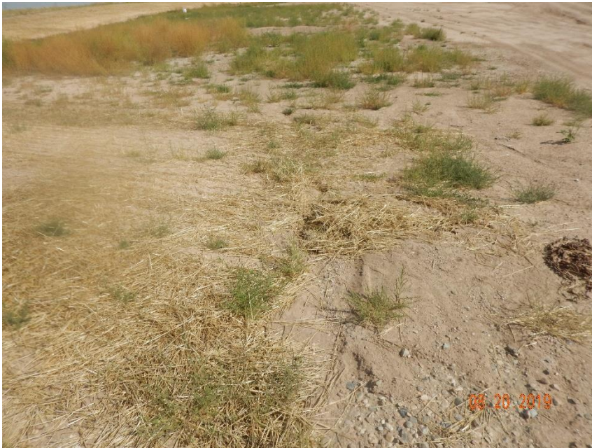
Photo 41: Photo taken from the southwest end of the pad, facing north. Photo shows stormwater runoff from the access road is beginning to cause erosion on the pad.
