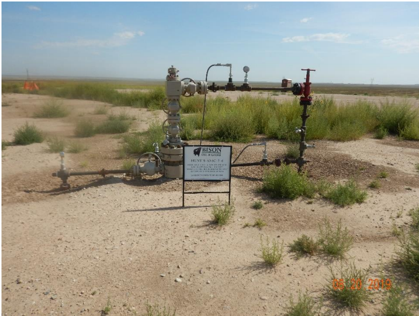
Photo 45: Photo taken from the Hunt 8-60 6C-5-6 well. Photo shows weed establishment on location and evidence of stormwater ponding at well. See comments under photo 42.
