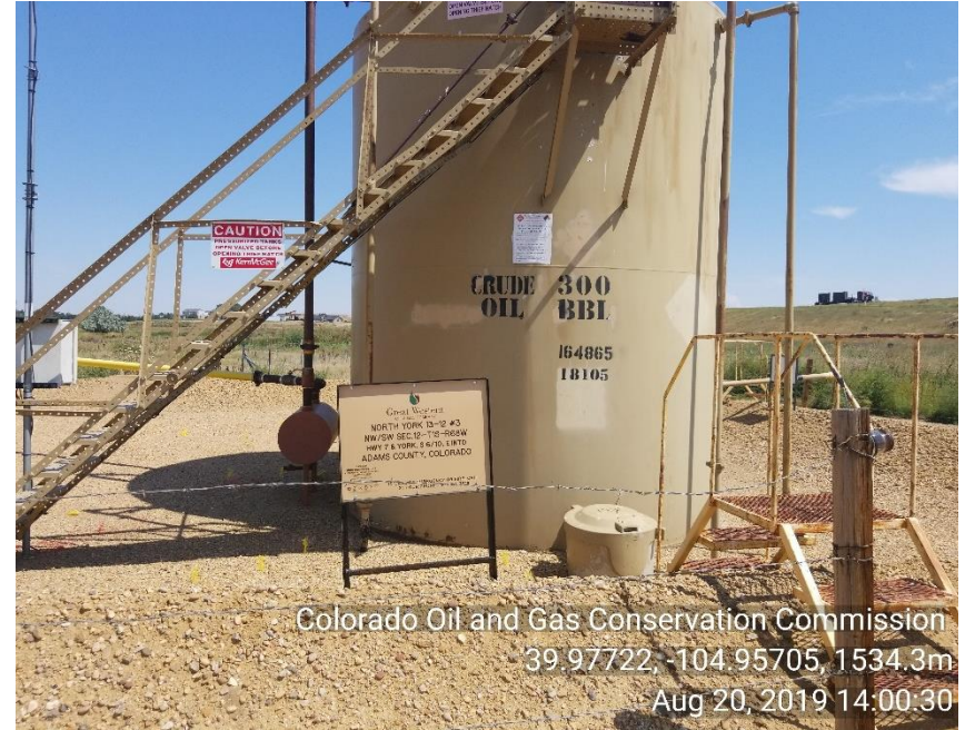
Photo 2 Crude oil tank placard has been replaced and tank appears to have been drained.
