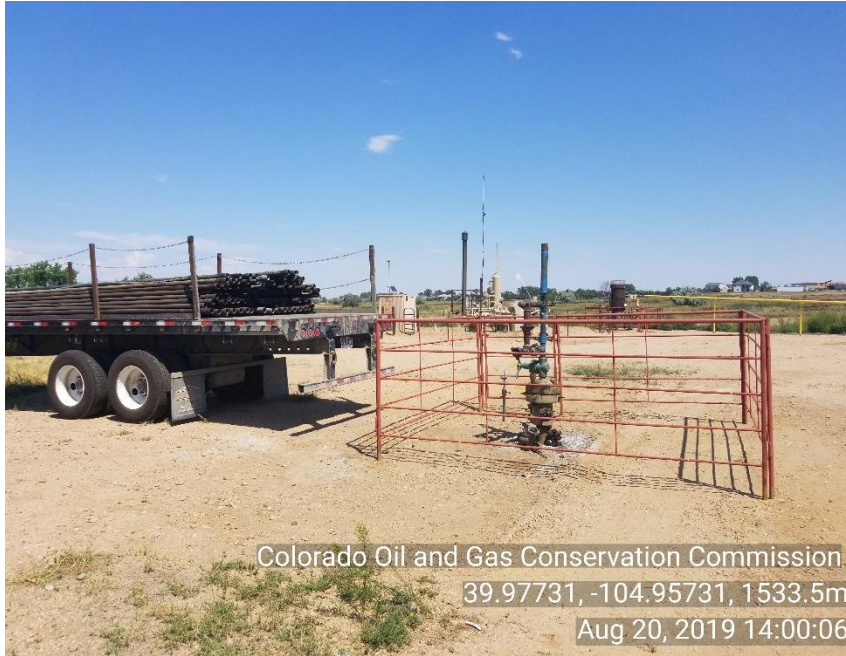
Photo 1 Well appears to be in the P&A process
