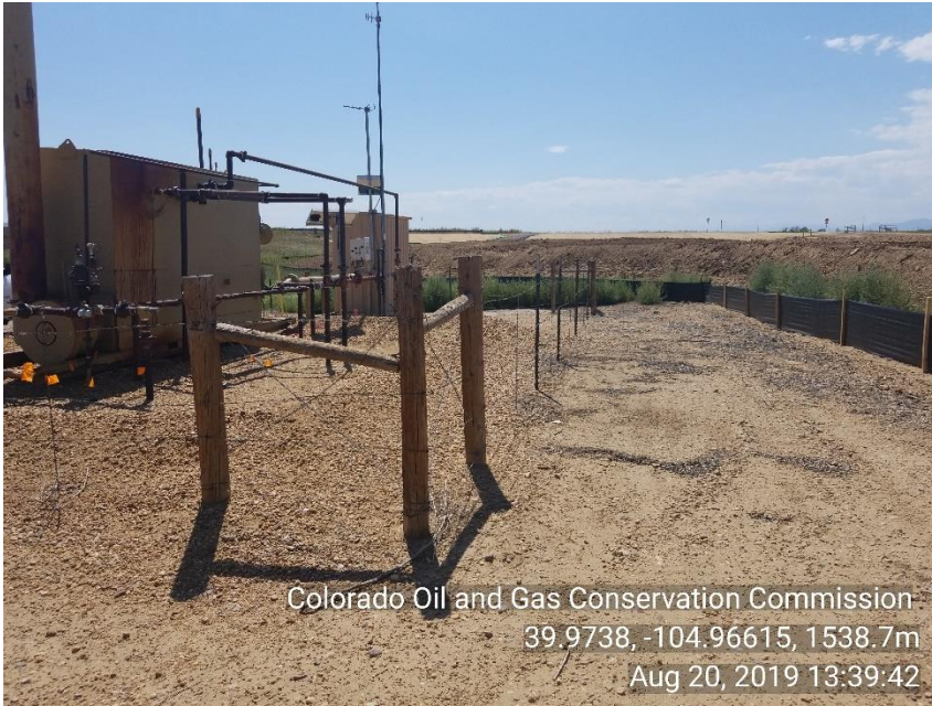
Photo 3 SEP. Trash around sep has been removed.
