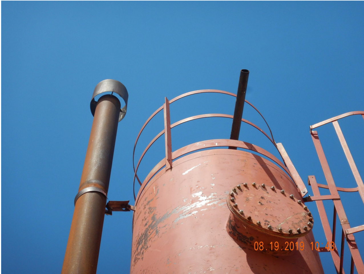
Photo 7. Photo taken of the heater treater stack. Photo illustrates Operator has failed to install wildlife intrusion mitigation device on top of the heater treater stack.
