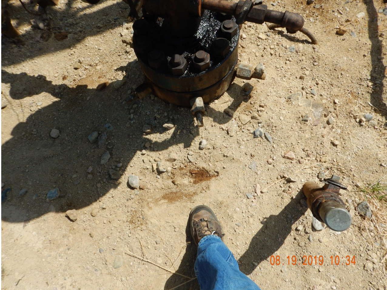
Photo 1. Photo taken of the wellhead. Wellhead appears to be leaking and has not been fixed since the previous inspection. Also, Operator has not properly treated or disposed of the oily waste in accordance with 907.e.; Operator has only put gravel on top of oily waste.
