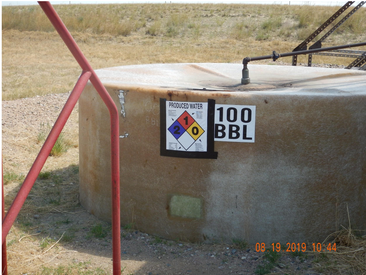
Photo 8. Photo taken of the production water tank on location. Operator has installed NFPA label.
