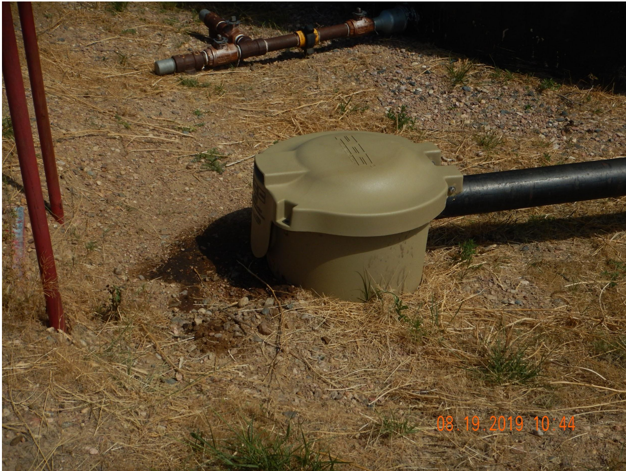
Photo 9. Photo taken from the load line bucket. Photo illustrates stained soil around bucket.
