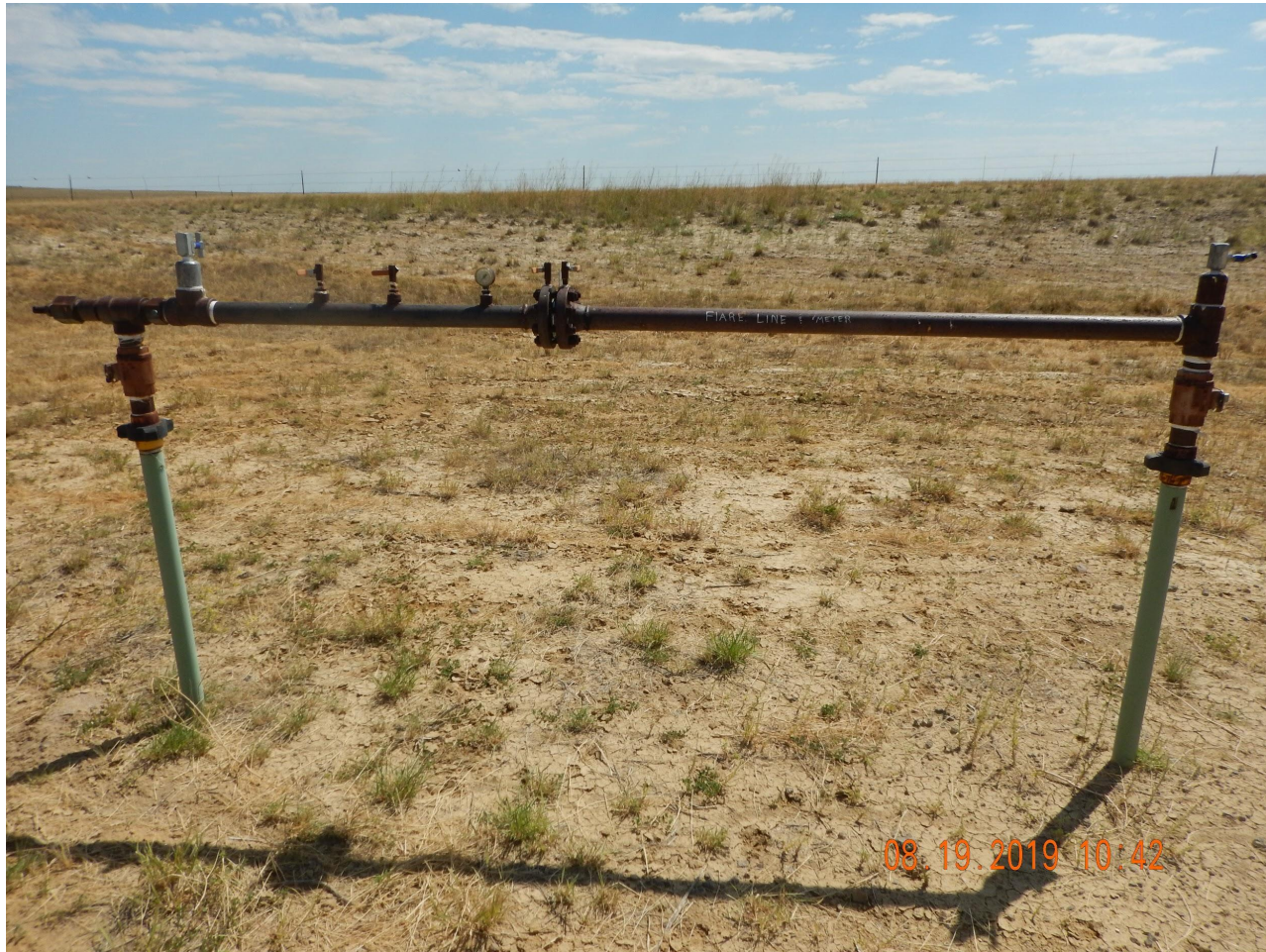
Photo 6. Photo taken from the north side of the treater shed, facing East. Photo illustrates unused meter run set with no meter.
