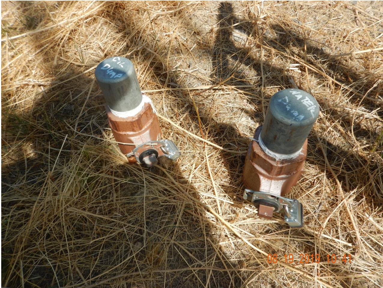
Photo 4. Photo taken from the north side of the treater shed. Photo illustrates that 2 of the risers have been locked out but not tagged out.
