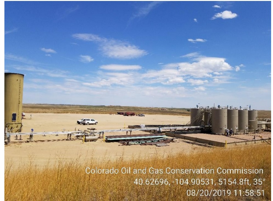
Photo 2 – Colorado Lakes Pad. Loc ID 449968. South looking North
