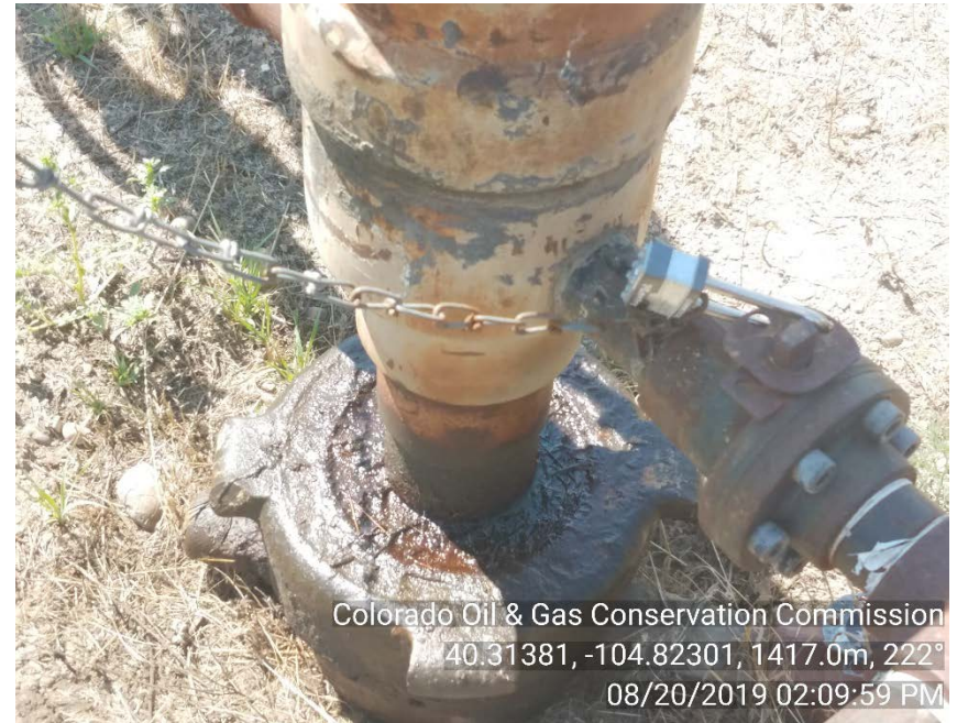
Bradenhead leak
