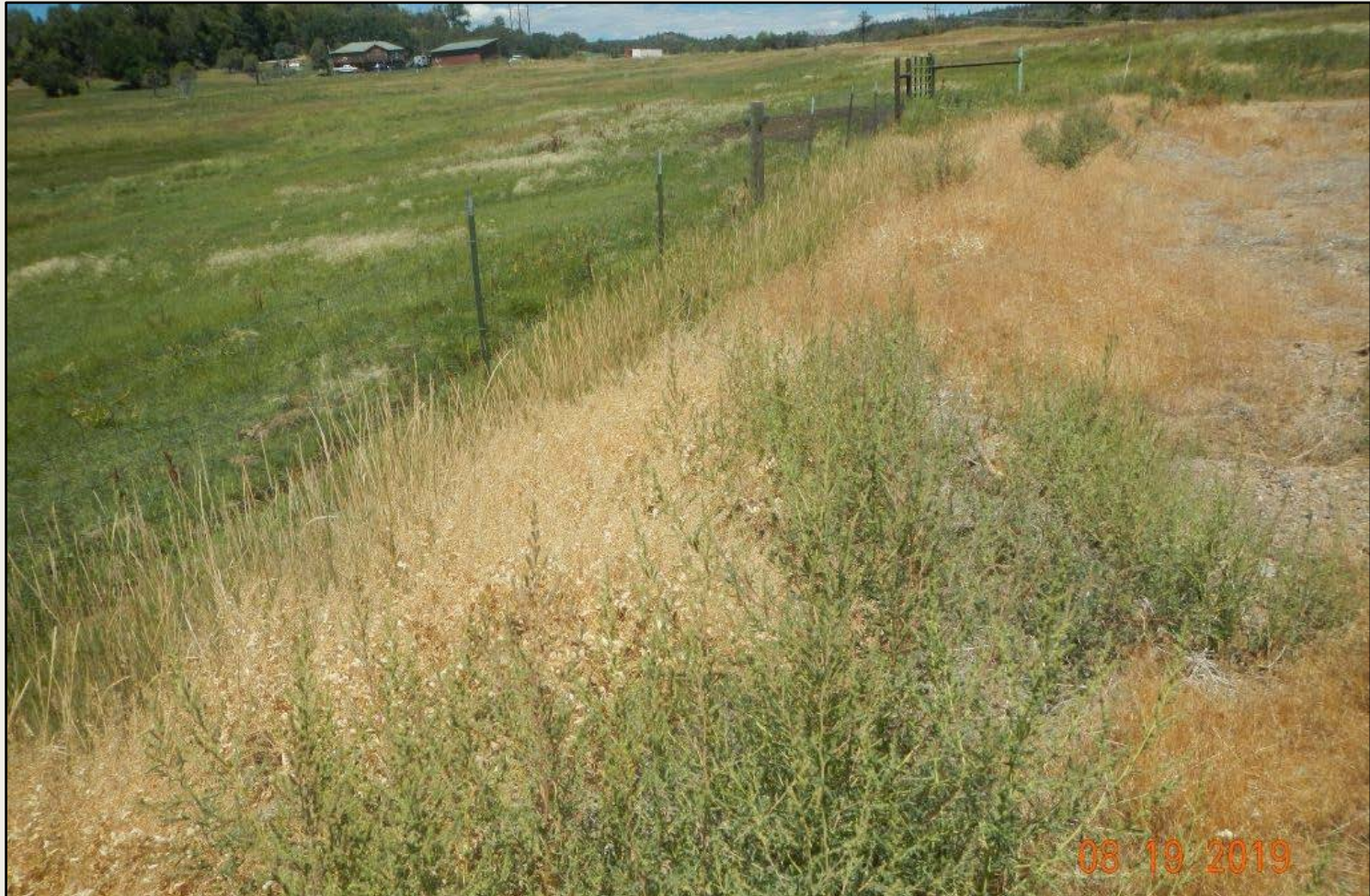
Photo 2. View of eastern fill slope facing northward.
