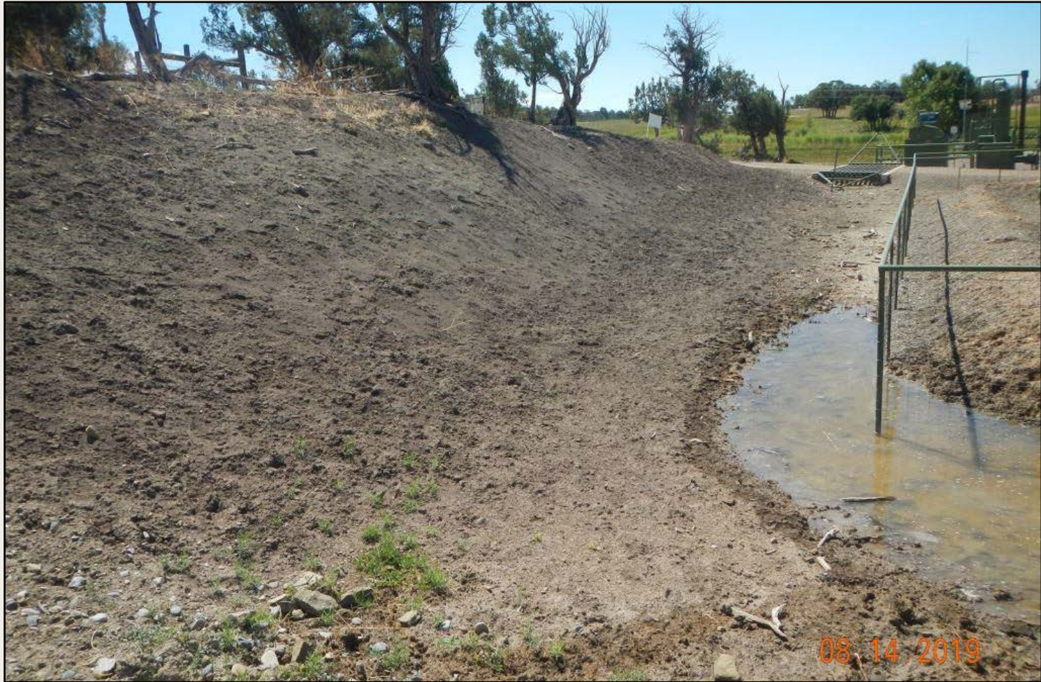
Photo 3. View of the eastern project area from the northeastern edge facing southward. Cut-slope is not stabilized.
