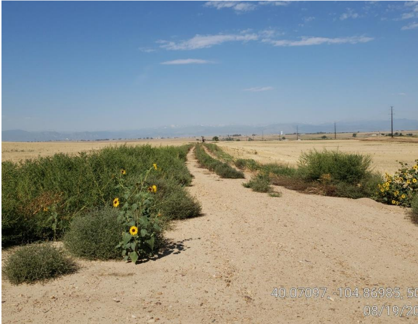
Photo #1 Tall weeds down center of Access Rd.
