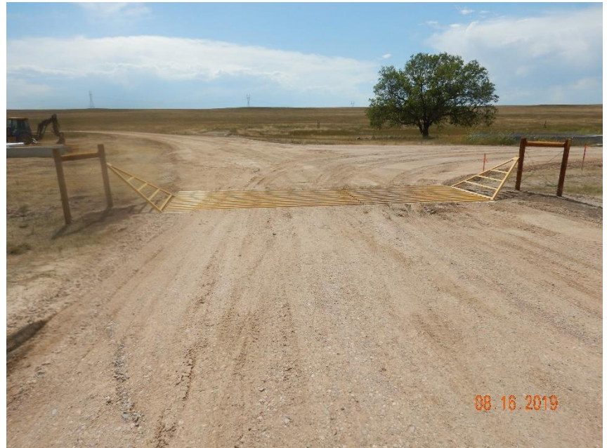
Photo 16: Photo taken from where the access road intersects with County Road 390, facing west. Photo shows vehicle tracking BMPs remain missing/insufficient at access road to motivate sediment transport from the disturbance areas (location/access road).
