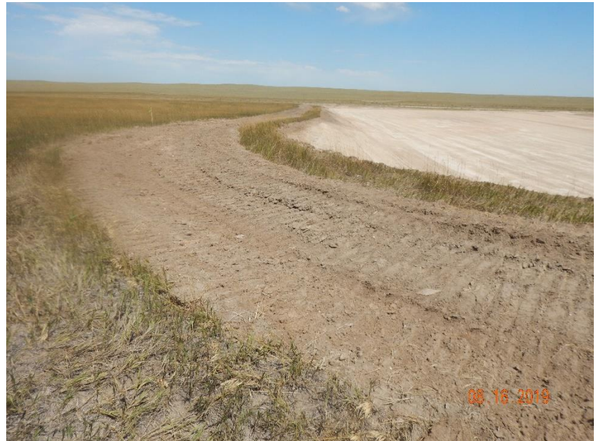
Photo 12: Photo taken from the northwest corner of the location, facing east. Photo shows section of perimeter stormwater diversion ditch that appear to be constructed in accordance with good engineering practices.
