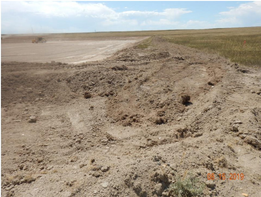
Photo 9: Photo taken from the sediment trap on the northeast corner of the location. See comments under photo 1. Photo also shows ditch on the northeast end of the location remains predominantly loose, unconsolidated/uncompacted material.
