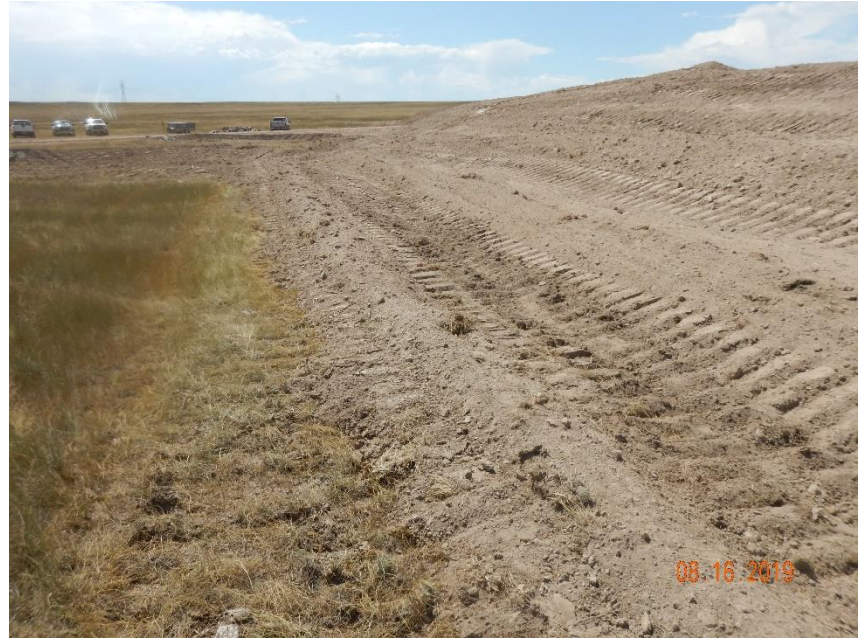
Photo 6: Photo shows stormwater diversion ditch on the southeastern perimeter of the location. Photo shows stormwater has not been constructed in accordance with good engineering practices and remains predominantly loose, unconsolidated/uncompacted material.
