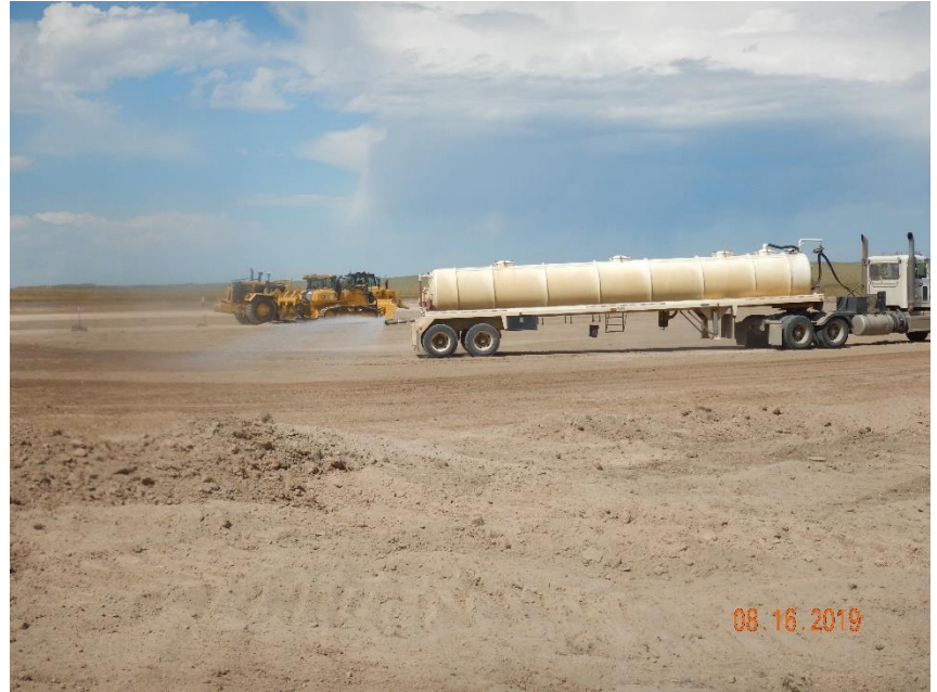
Photo 14: Photo shows operator using a water truck to mitigate fugitive dust from the location.
