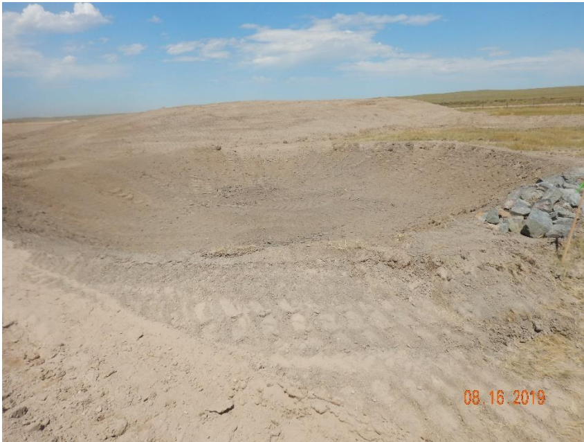
Photo 1: Photo taken from the south end of the location, facing east. Photo shows 1 of the 4 sediment traps on the location. Sediment trap has been enlarged, however, sediment trap has not been constructed in accordance with good engineering practices and is missing sufficient inlet and outlet protection. Coarse rock aggregate used appears too large to slow stormwater discharge. No geotextile lining has been installed beneath the rip-rap
