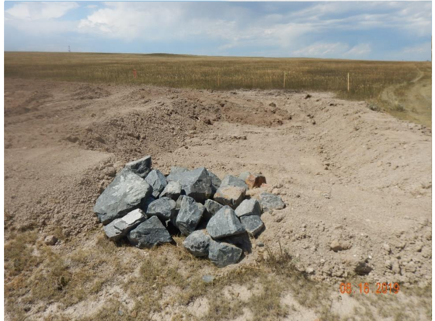
Photo 8: Photo of sediment trap on the northeast end of the location. Photo shows sediment trap has not been constructed in accordance with good engineering practices.
