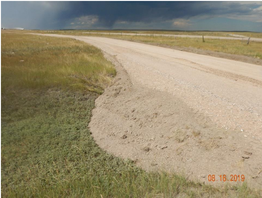
Photo 15: Photo taken from section of access road that was constructed over a drainage. Photo shows no BMPs have been installed to prevent stormwater ponding, and allow for water movement under access road .
