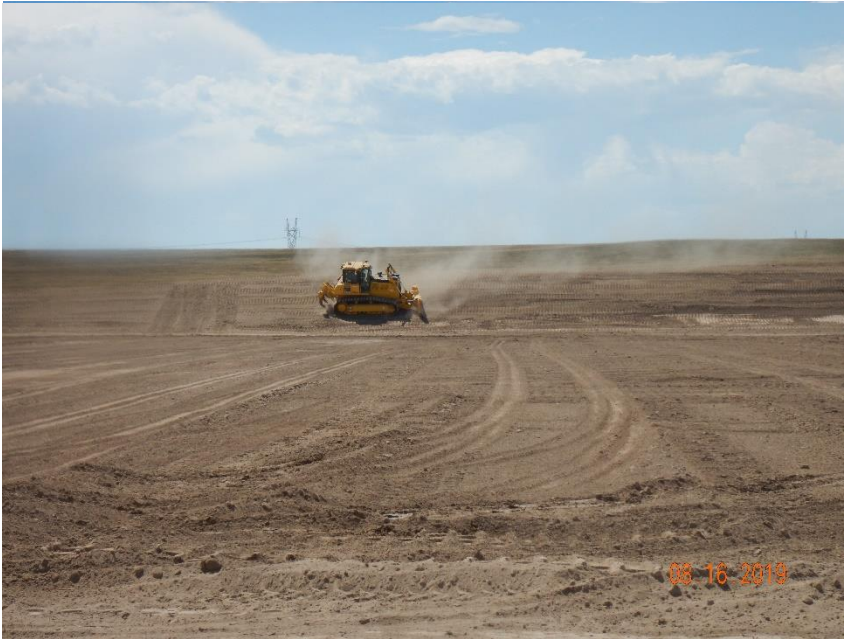
Photo 7: Photo taken from the east end of the location, facing west. Photo shows operator has installing surface roughening (tracking) on slopes. Tracking has been installed along the contour of the slopes, rather than up and down.
