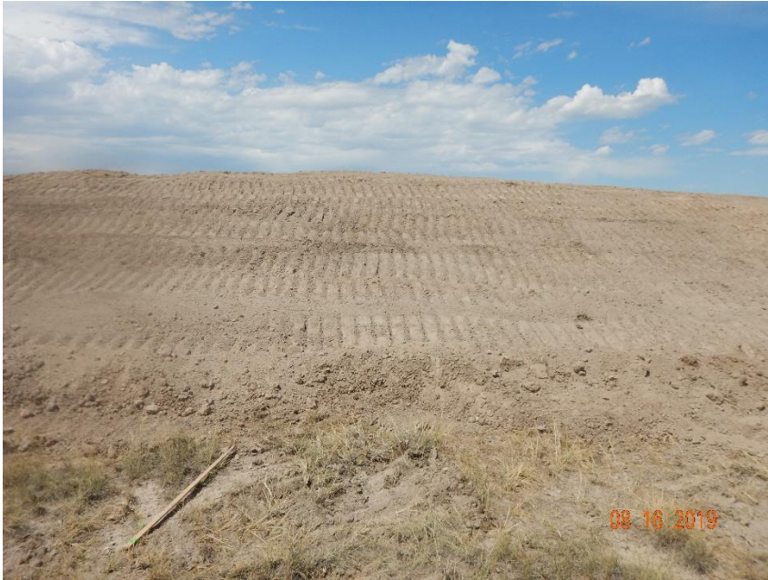
Photo 3: Photo taken from the topsoil stockpile on the south end of the location. Photo shows operator has installed surface roughening (tracking) on slopes. Tracking has been installed along the contour of the slopes, rather than up and down.
