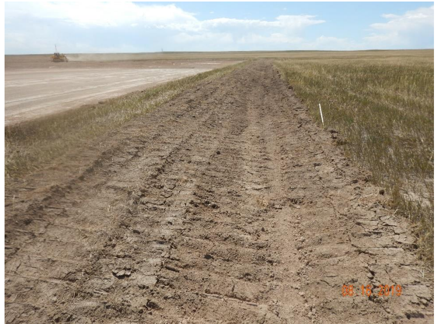
Photo 10: Photo taken from the north end of the location, facing west. Photo shows section of perimeter stormwater diversion ditch that appear to be constructed in accordance with good engineering practices.
