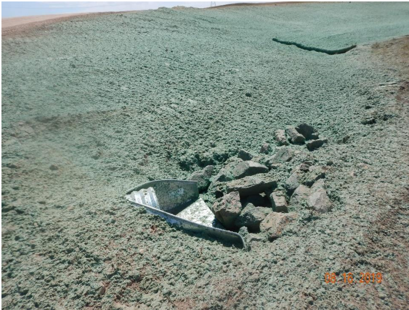
Photo 3: Photo of culvert at the north end of the location. Photo shows armorment/stormwater protection remains missing/insufficient.
