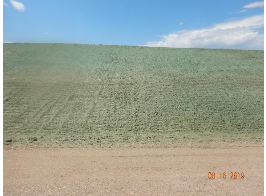
Photo 12: Photo taken from the south end of the location, facing south. Photo shows tracking has been re-installed up and down the slopes and is now being used in conjunction with a tackifier.
