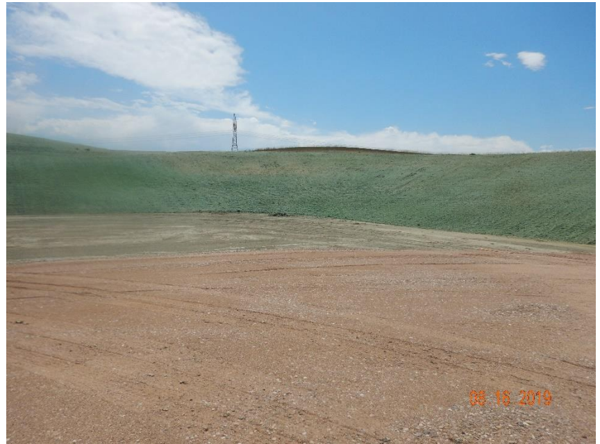
Photo 14: Photo taken from the southwest end of the location, facing southwest. Photo shows tracking has been re-installed up and down the slopes and is now being used in conjunction with a tackifier.
