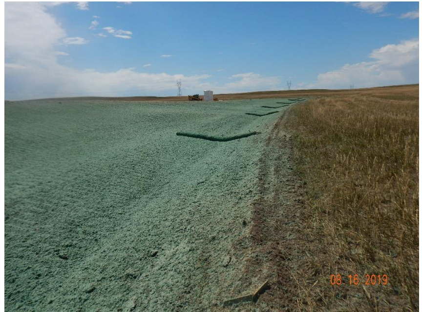
Photo 4: Photo taken from the north end of the location, facing west. Photo shows ditch appear to have been installed in accordance with good engineering practices; ditch appears sufficiently consolidated/compacted. Operator has installed a tackifier as an additional stabilization within ditch.
