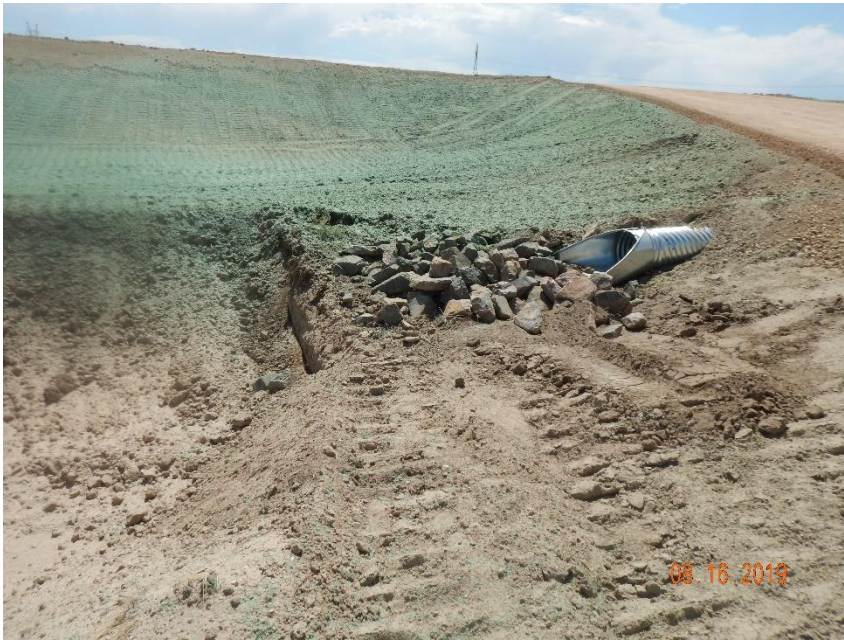
Photo 5: Photo of culvert at the north end of the location. Photo shows armoring/stormwater protection remains missing/insufficient. Photo also shows sediment trap has not been constructed in accordance with good engineering practices and is missing sufficient inlet and outlet protection.
