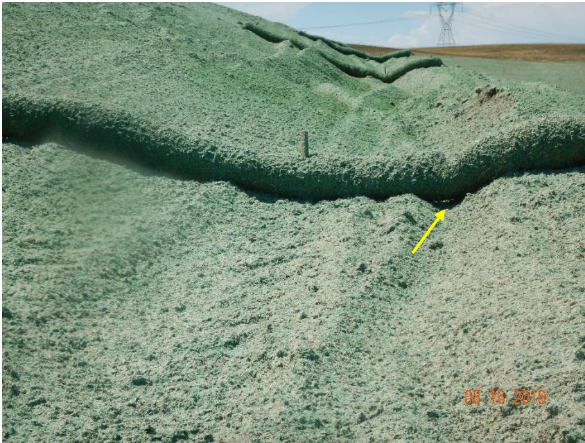
Photo 13: Photo taken from the ditch at base of the soil stockpile on the south end of the location. Photo shows Operator has selected/placed straw wattles within the ditch of the location. Wattles appear to have been placed as a "Velocity Check". Straw wattles have not been installed in accordance with good engineering practices. Wattles are required to be trenched and back-filled in order to be in proper functioning condition. Insufficient trenching/backfilling will result in degradation to the ditch due to stormwater cutting and passing beneath the wattle. Arrow pointing at daylight observed from under the wattle.
