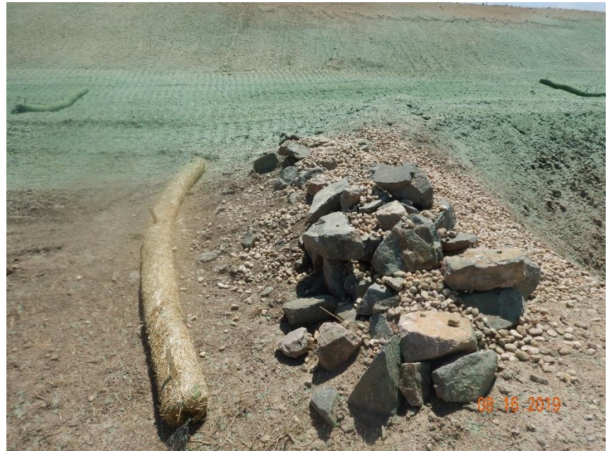
Photo 6: Photo taken from the sediment trap on the north end of the location. Photo shows sediment trap has not been constructed in accordance with good engineering practices and is missing sufficient inlet and outlet protection. Additional smaller sized rip-rap has been placed at outlet in conjunction with the larger aggregate material observed in the previous inspection however, it does not appear as though operator has installed a geotextile lining beneath the coarse aggregate and rip-rap. Wattle has only been placed and staked upon surface, and has not been trenched/backfilled in accordance with good engineering practices.
