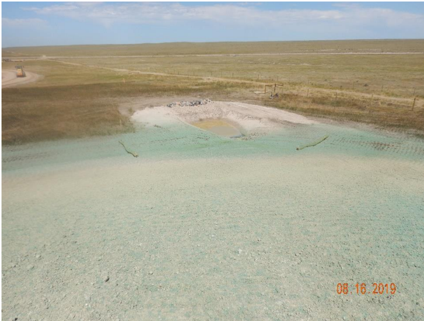
Photo 1: Photo taken from the north east end of the location, facing northeast. Photo shows 1 of the 4 sediment traps on the location. Photo also shows tracking has been re-installed up and down the slopes and is now being used in conjunction with a tackifier.
