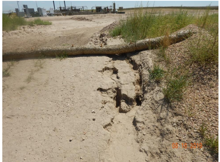
Photo 12: See comments under photo 11. Photo shows insufficient inlet protection (BMP not installed in accordance with good engineering practices) has contributed to the failure of the sediment trap.
