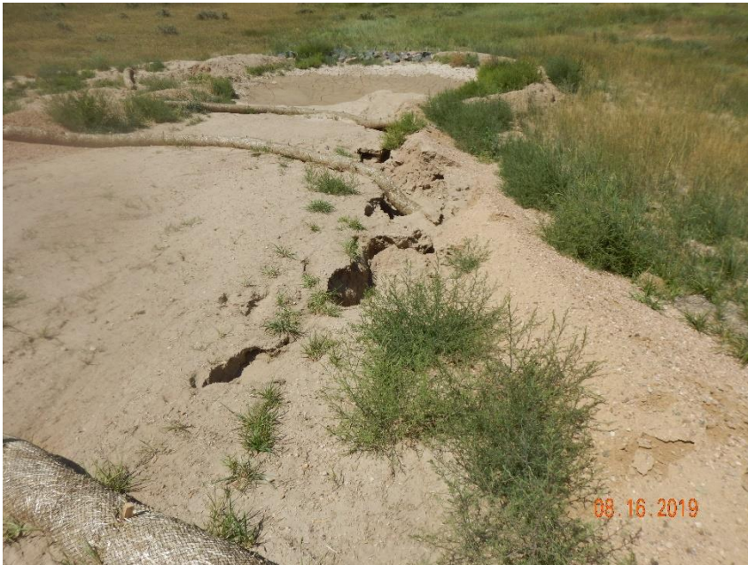
Photo 11: Photo taken from the northwest corner of the location. Photos 11-19 show the Stormwater sediment traps constructed on location have not been constructed in accordance with good engineering practices. BMPs were not constructed to an appropriate size for the site's conditions, or with sufficient inlet/outlet and slope protection. As a result, stormwater has degraded the trap and BMP is no longer in proper functioning condition. Sediment transport off location evident.
