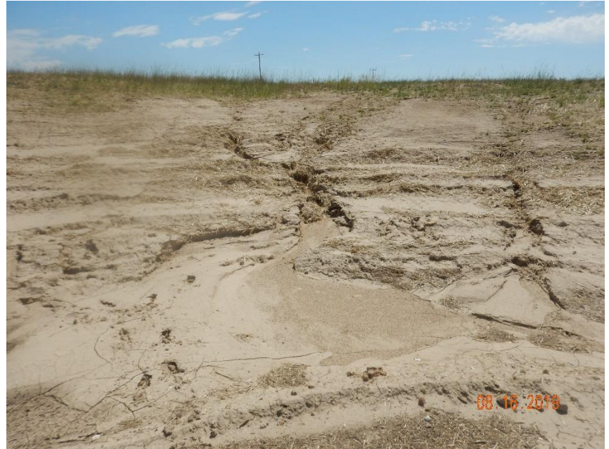
Photo 4: Photo taken from the southeast end of the location. See comments under photo 1. Photo also shows ditch remains filled with sediment and is not in proper functioning condition.
