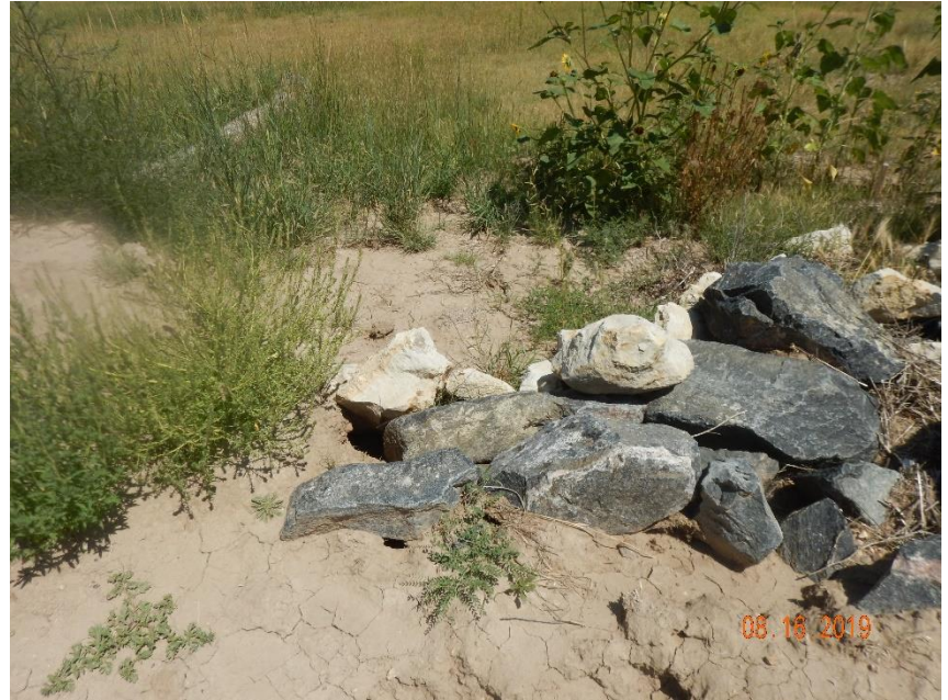
Photo 22: Continued from photo 21. Photo shows insufficient outlet protection (BMP not installed in accordance with good engineering practices) has contributed to the failure of the sediment trap and allowed for sediment discharge from location.
