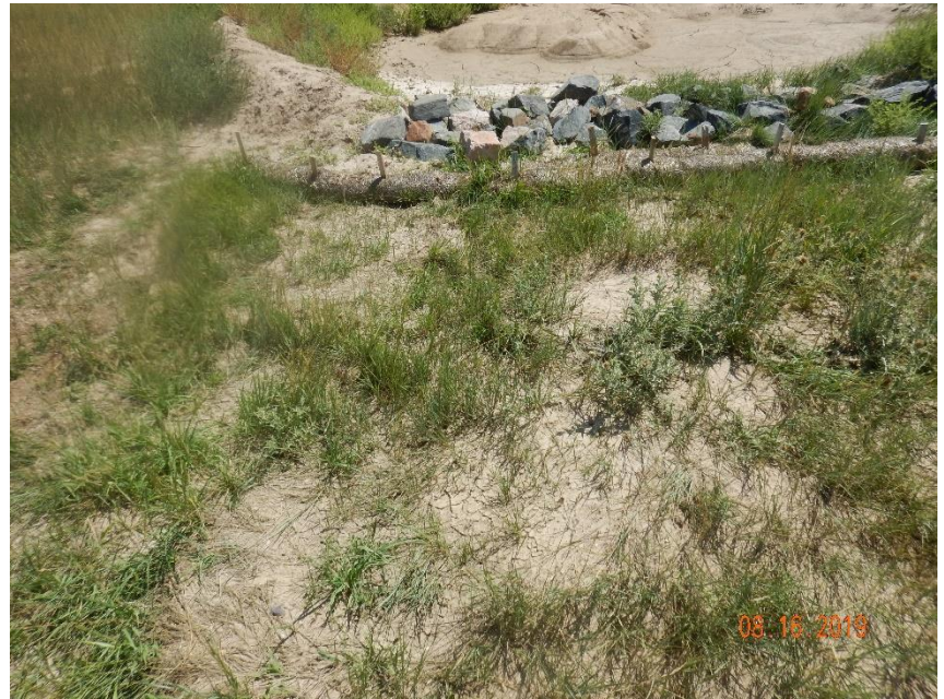
Photo 18: Continued from photo 16. Photo shows insufficient outlet protection (BMP not installed in accordance with good engineering practices) has contributed to the failure of the sediment trap and allowed for sediment discharge from location.
