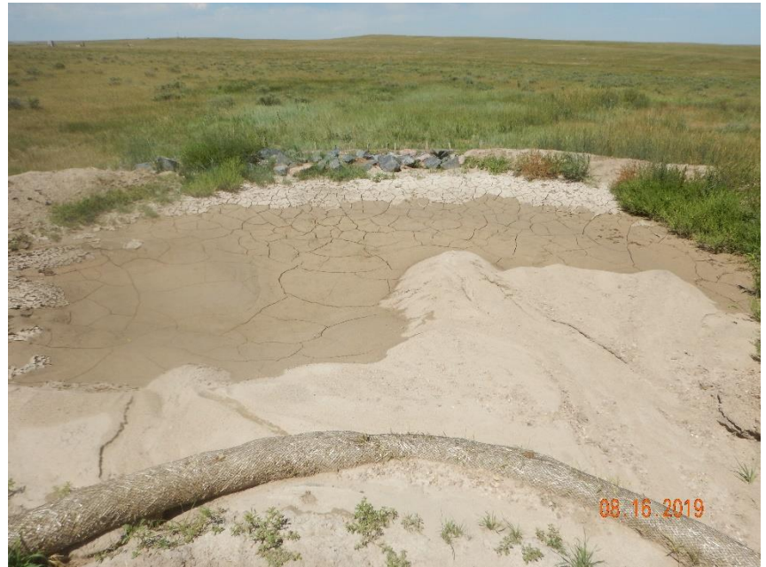
Photo 14: See comments under photo 11. Photo shows sediment has filled the trap. BMP was not installed in accordance with good engineering practices and is no longer in proper functioning condition.
