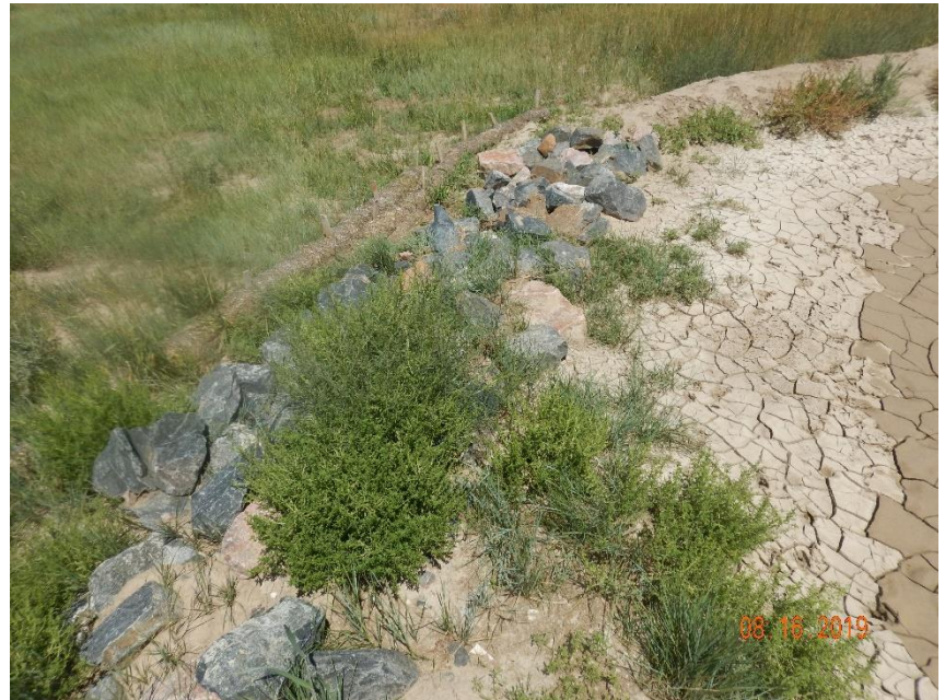
Photo 16: See comments under photo 11. Photo shows insufficient outlet protection (BMP not installed in accordance with good engineering practices) has contributed to the failure of the sediment trap and allowed for sediment discharge from location.
