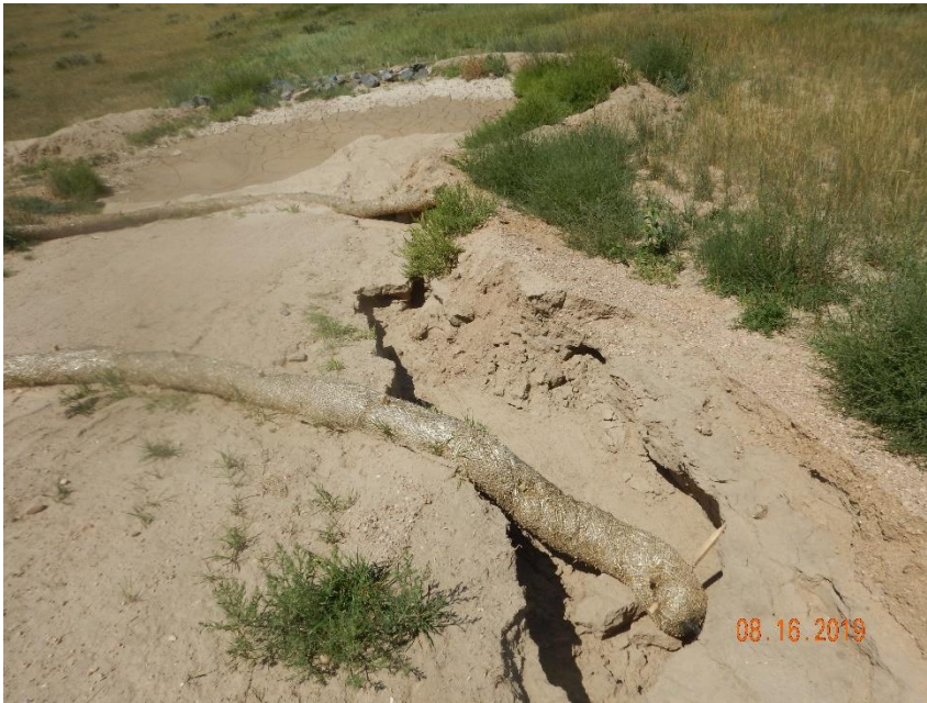
Photo 13: See comments under photo 11. Photo shows insufficient inlet protection (BMP not installed in accordance with good engineering practices) has contributed to the failure of the sediment trap.
