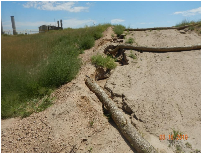
Photo 15: See comments under photo 11. Photo shows sediment has filled the trap. BMP was not installed in accordance with good engineering practices and is no longer in proper functioning condition.
