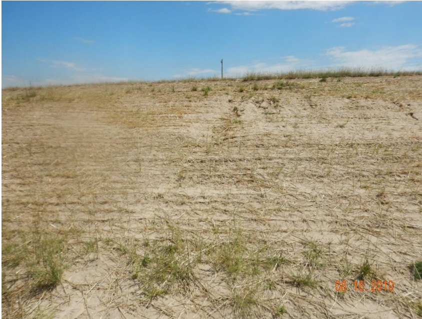
Photo 1: Photo taken from the east end of the location, facing east. Photo shows erosion degradation on slopes. Operator has failed to conduct sufficient and ongoing stormwater management and monitoring; Operator has failed install or maintain sufficient stormwater and erosion control BMPs based on the sites conditions and in accordance with good engineering practices.
