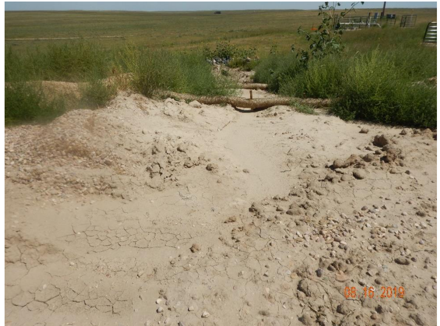
Photo 20: Photo taken from the sediment trap on the northeast end of the location. Photos 20- 22 show the Stormwater sediment traps constructed on location have not been constructed in accordance with good engineering practices. BMPs were not constructed to an appropriate size for the site's conditions, or with sufficient inlet/outlet and slope protection. As a result, stormwater has degraded the trap and BMP is no longer in proper functioning condition. Sediment transport off location evident.
