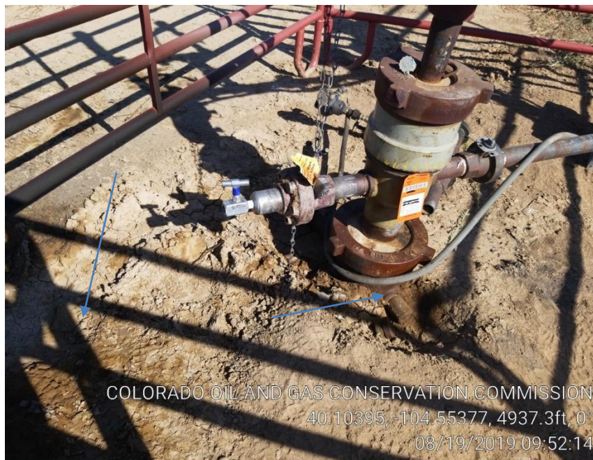
Pic 5 stained soil/mechanical conditions
