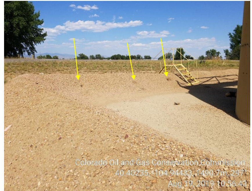
Photo 6: Holes in berm wall
