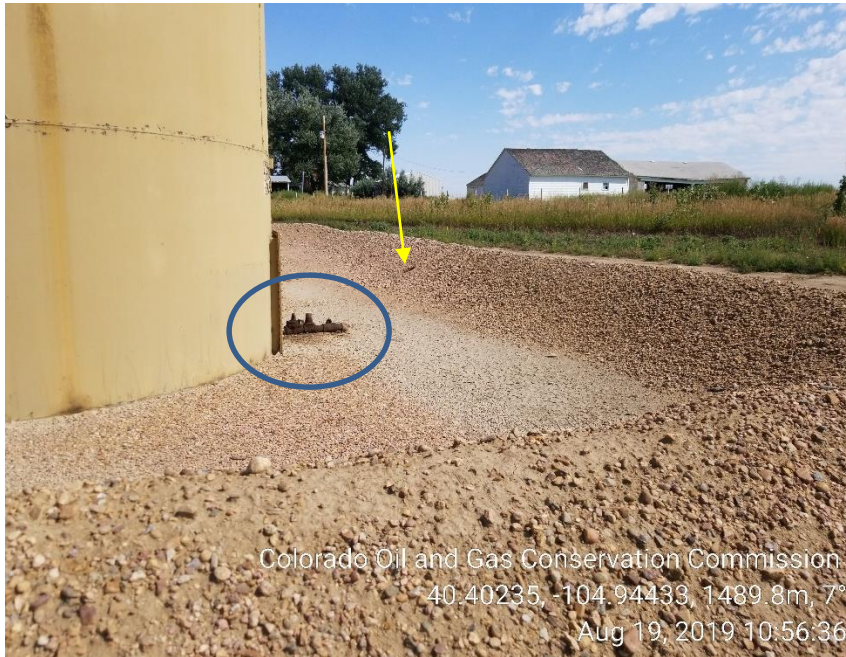
Photo 5: Stained soil/ Hole in berm
