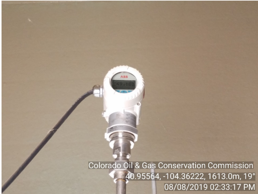
Photo #3 Simba 1-06 SWD UIC - Wellsite Tbg. Press: 49# Injecting
