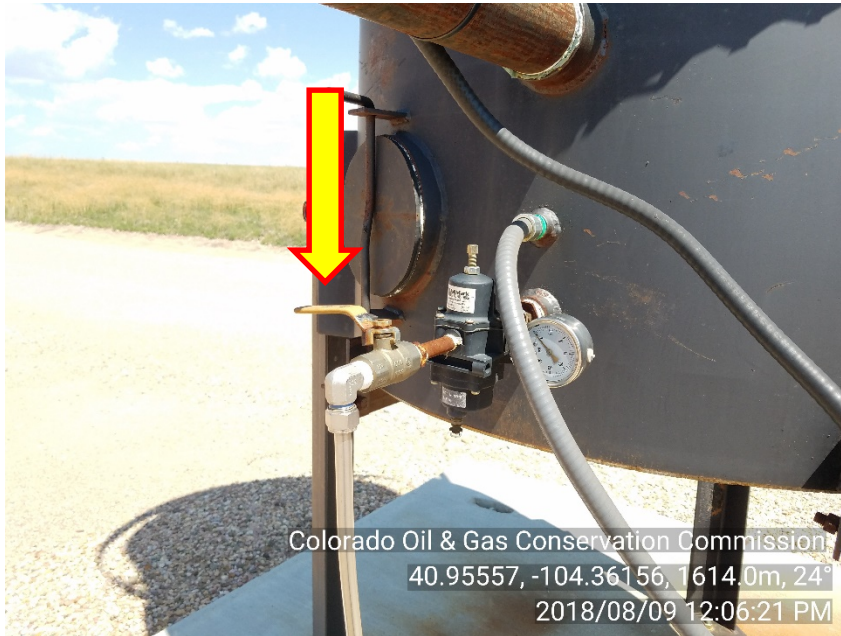
Photo #15 Simba 1-06 SWD UIC – Disposal Facility ECD: pilot supply gas off prior insp.
