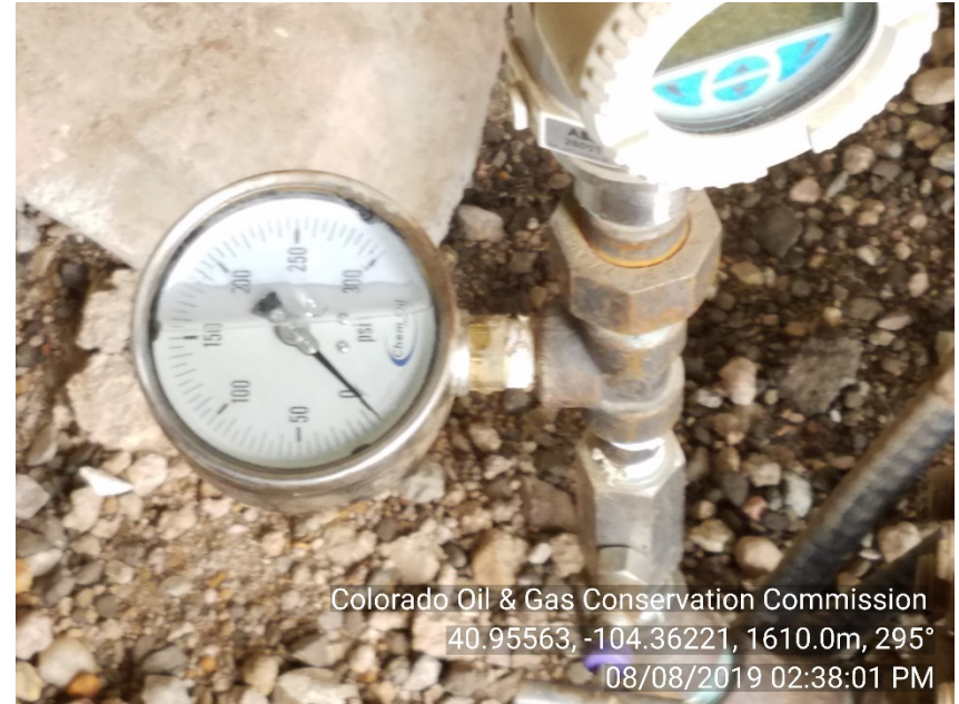
Photo #4 Simba 1-06 SWD UIC - Wellsite Csg Press: 0#
