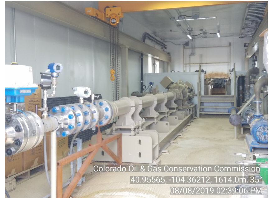
Photo #6 Simba 1-06 SWD UIC - Disposal Facility Injection pump Active operation / Injecting
