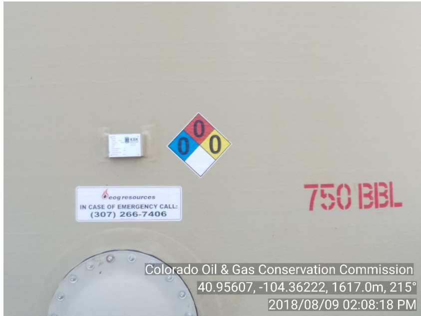
Photo #7 Simba 1-06 SWD UIC – Disposal Facility Produced H2O Tanks Incorrect NFPA placards prior insp.
