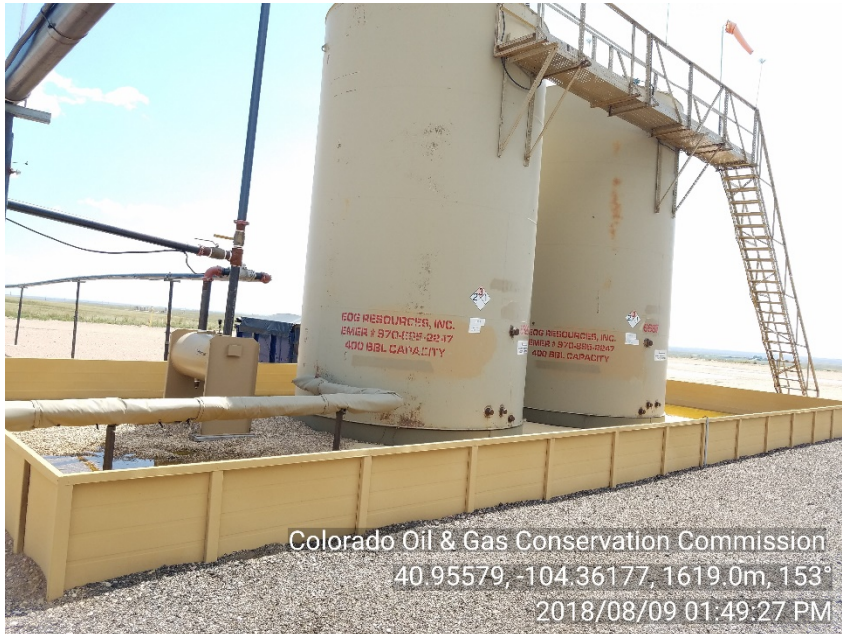
Photo #11 Simba 1-06 SWD UIC – Disposal Facility Crude Oil Tanks Contents NOT posted prior insp.
