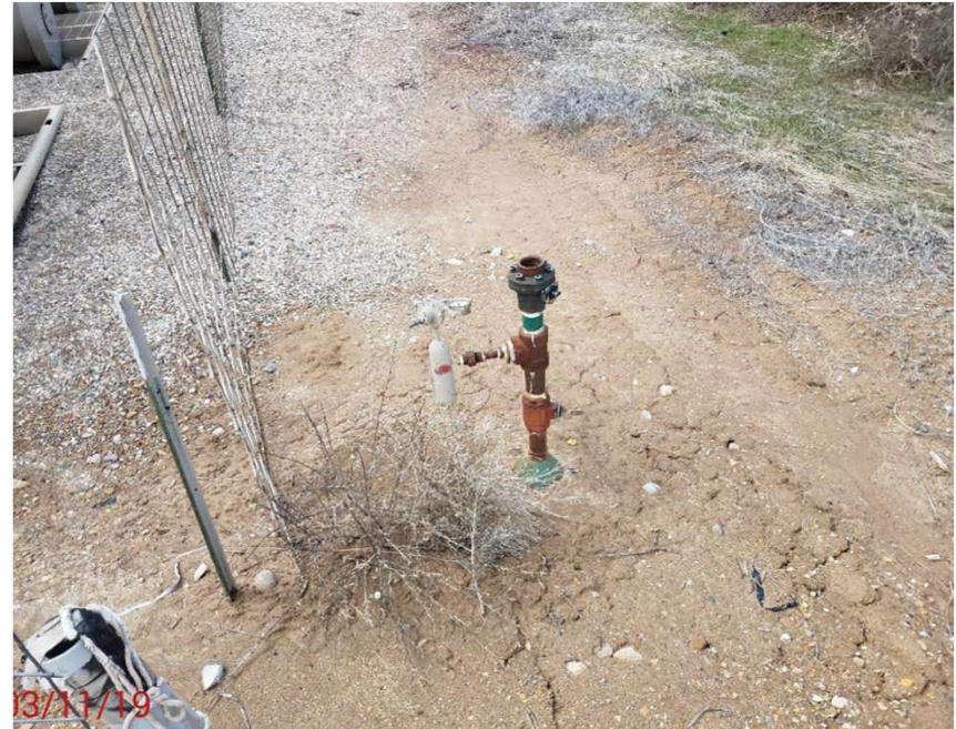
4 Previous inspection photo of flow line
