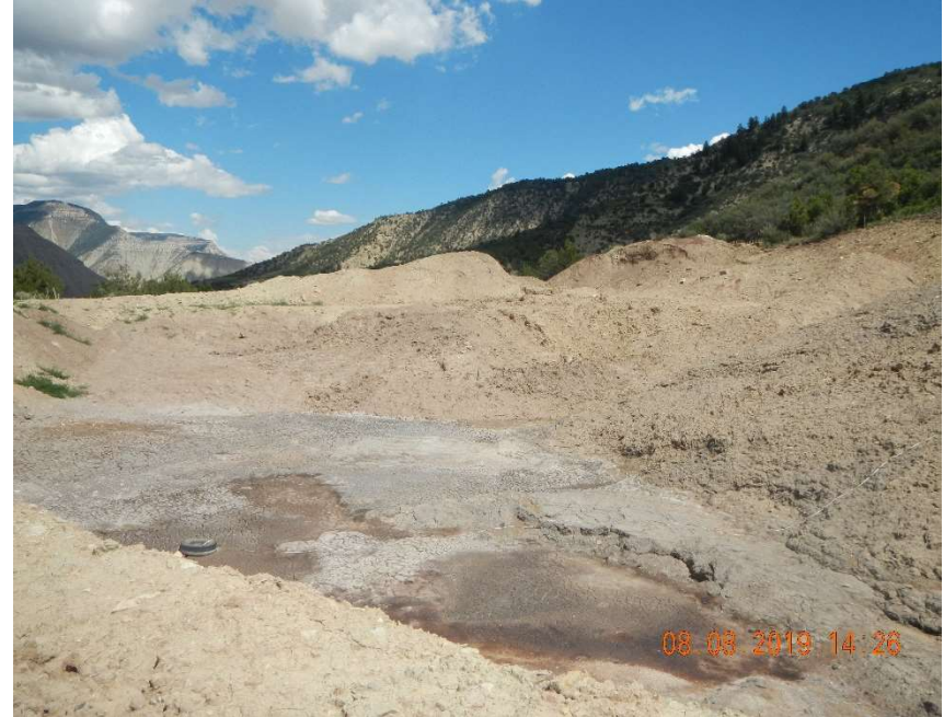
Photo #4 - View of cuttings trench looking southeast. Red / brown / dark brown soil in bottom of the trench is drilling mud.
