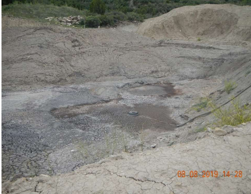
Photo #3 – View of cuttings trench looking southwest. Red / brown / dark brown soil in bottom of the trench is drilling mud.
