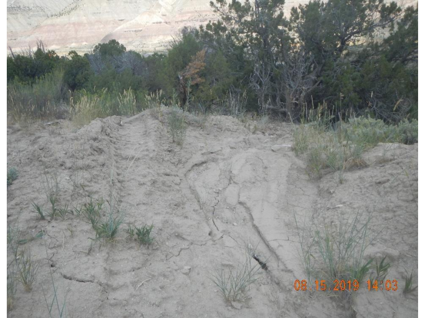
Overwhelmed and damaged check dam at entrance.
