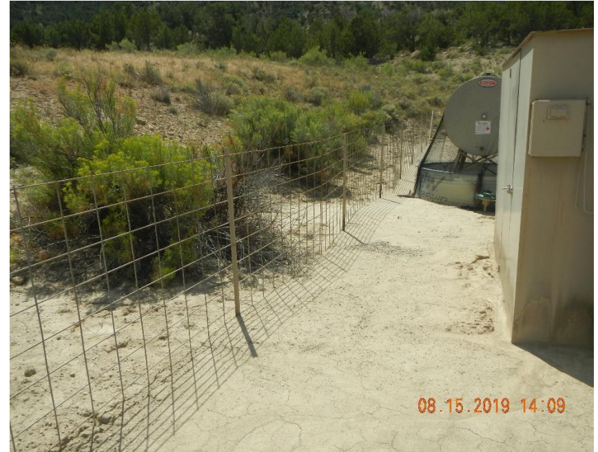
Sediment gathering around dehydrator.
