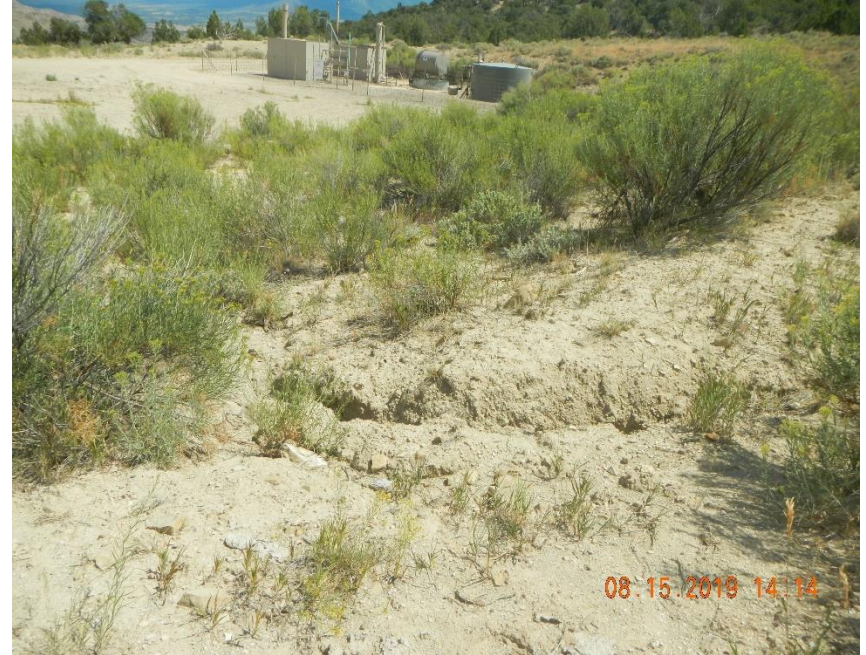
Breach of ditch wall.
