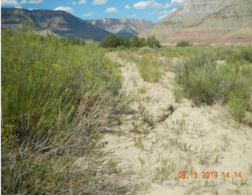
Diversion ditch full of sediment and breach of ditch wall.
