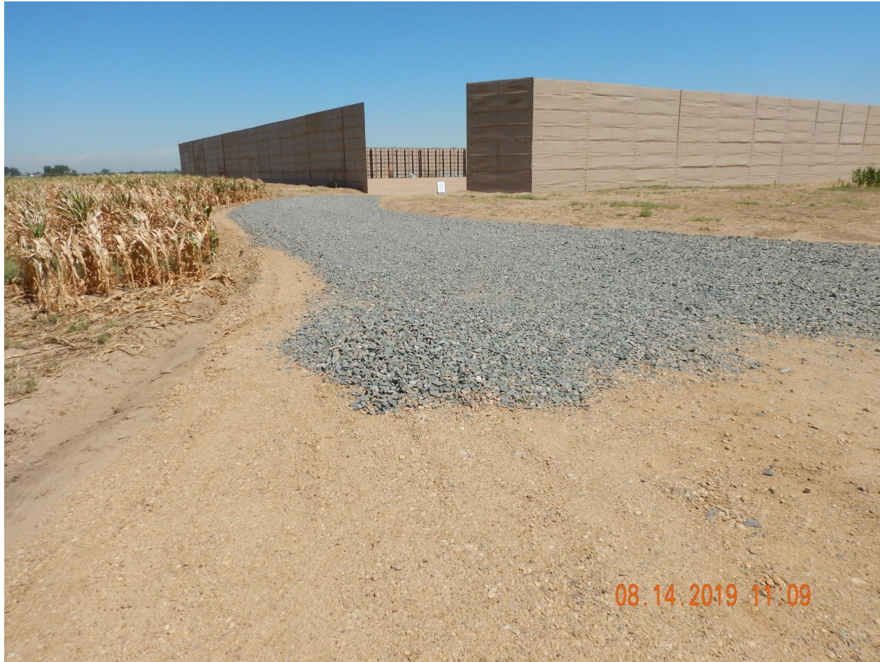
Photo 1. Photo taken from the entrance of Location, facing Northeast. Photo illustrates a vehicle tracking device BMP.
