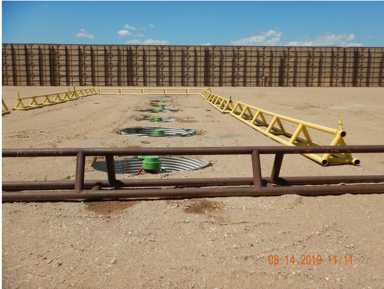
Photo 4. Photo taken from the central Location, facing West. Photo illustrates eight wells have spud the surface hole. Notification to run and cement casing was received in mid-July.
