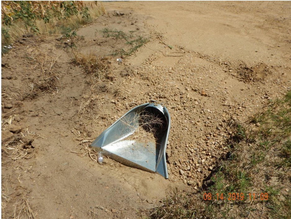
Photo 2. Photo taken from the entrance of Location, facing East. Photo illustrates a culvert installed along the roadside ditch. Operator shall stabilize both the inlet and outlet of the culvert.
