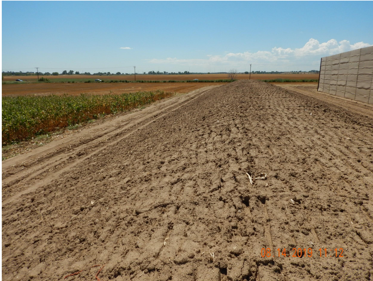
Photo 5. Photo taken from the eastern Location, facing South. Photo illustrates the topsoil stockpile which has been temporarily stabilized with equipment tracking.
