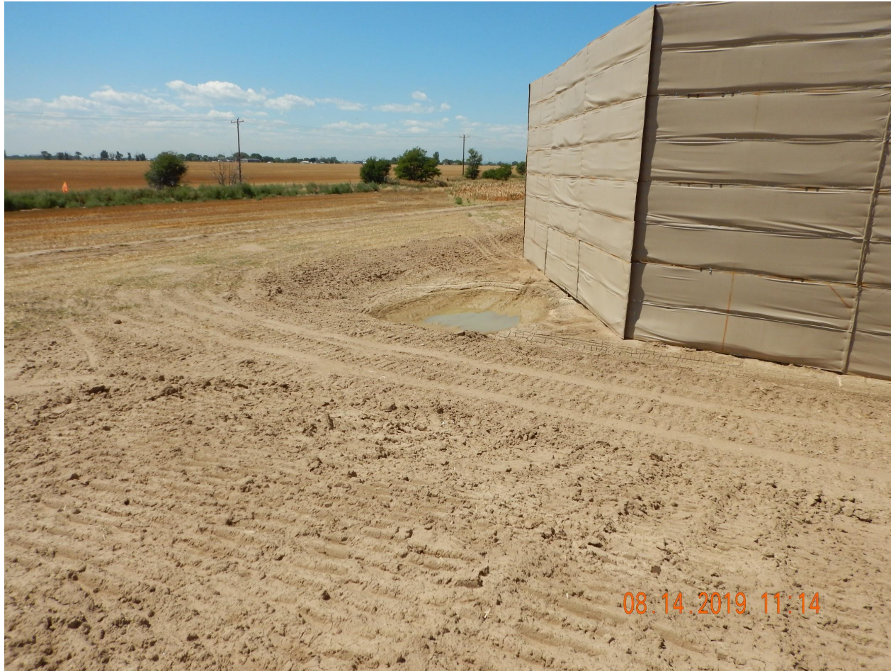
Photo 6. Photo taken from the southeastern Location, facing Southwest. Photo illustrates the well location and retention area which is all within a cut area. A ditch and berm BMP has also been installed along the outer perimeter of the location.
