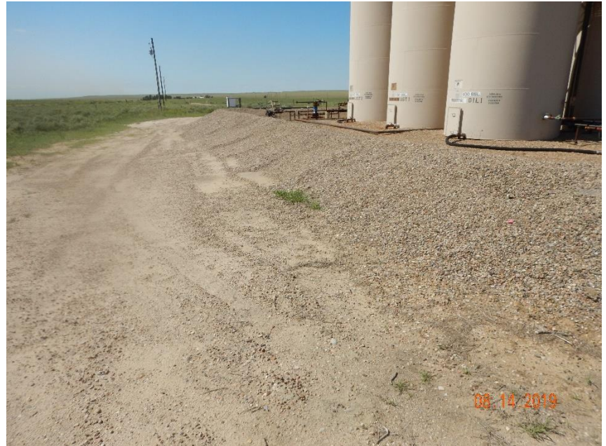
Photo 12: Photo taken from the east end of the tank battery, facing south. Photo shows vegetation has been removed from the berms.
