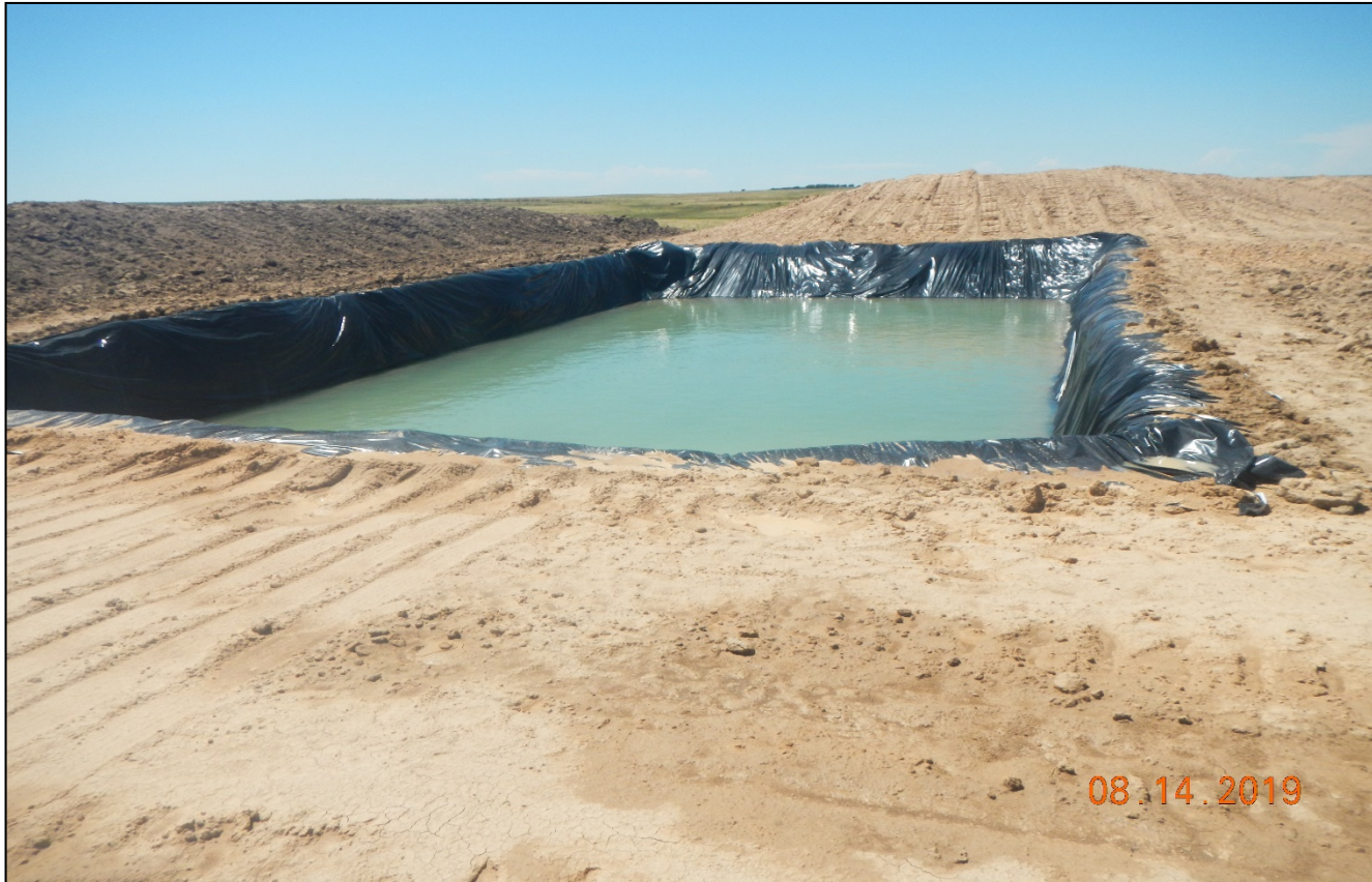
Photo 4. There is a lined pit filled with water.
