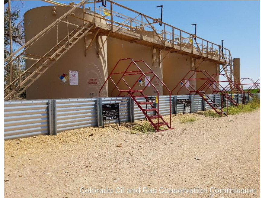
Photo 2: Centralized Tank Battery
