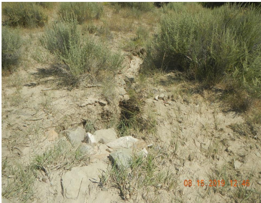
Erosion of check dam outlet.
