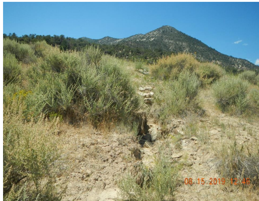
Erosion of check dam outlet.
