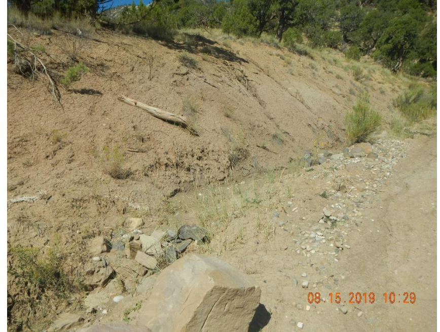
Sediment build up in road ditch.
