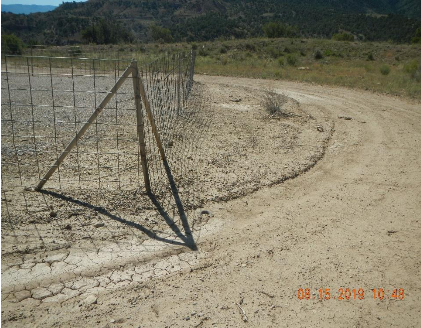
2 unmarked deadmen at S.W. corner of tank fence.
