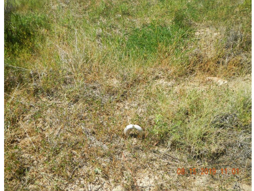
1 unmarked deadman off N.E. corner of location
