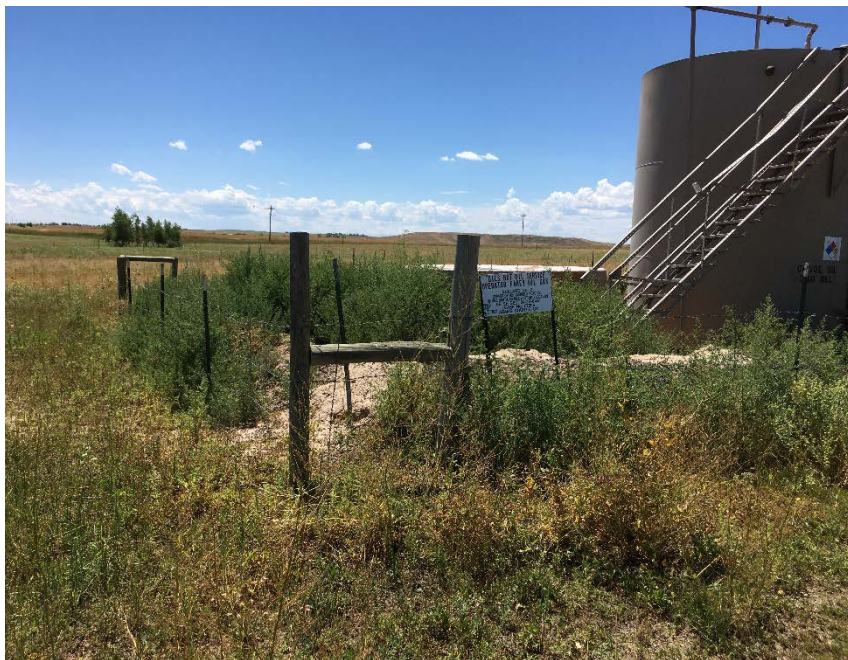
Tank Battery showing 1 – 300 BBL crude oil tank and 1 – 100 BBL produced water. Photo looking south. Very weedy.
