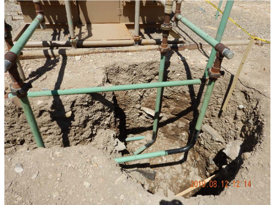
Photo #16 – Moist soil inside of northern end of excavation.
