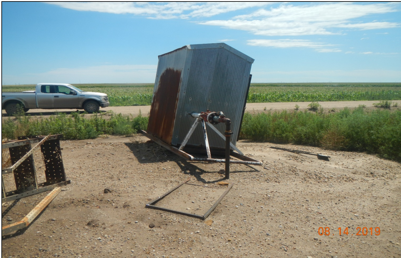
Photo 4. The meter shed does not appear to be stable and is leaning over which is a safety concern.
