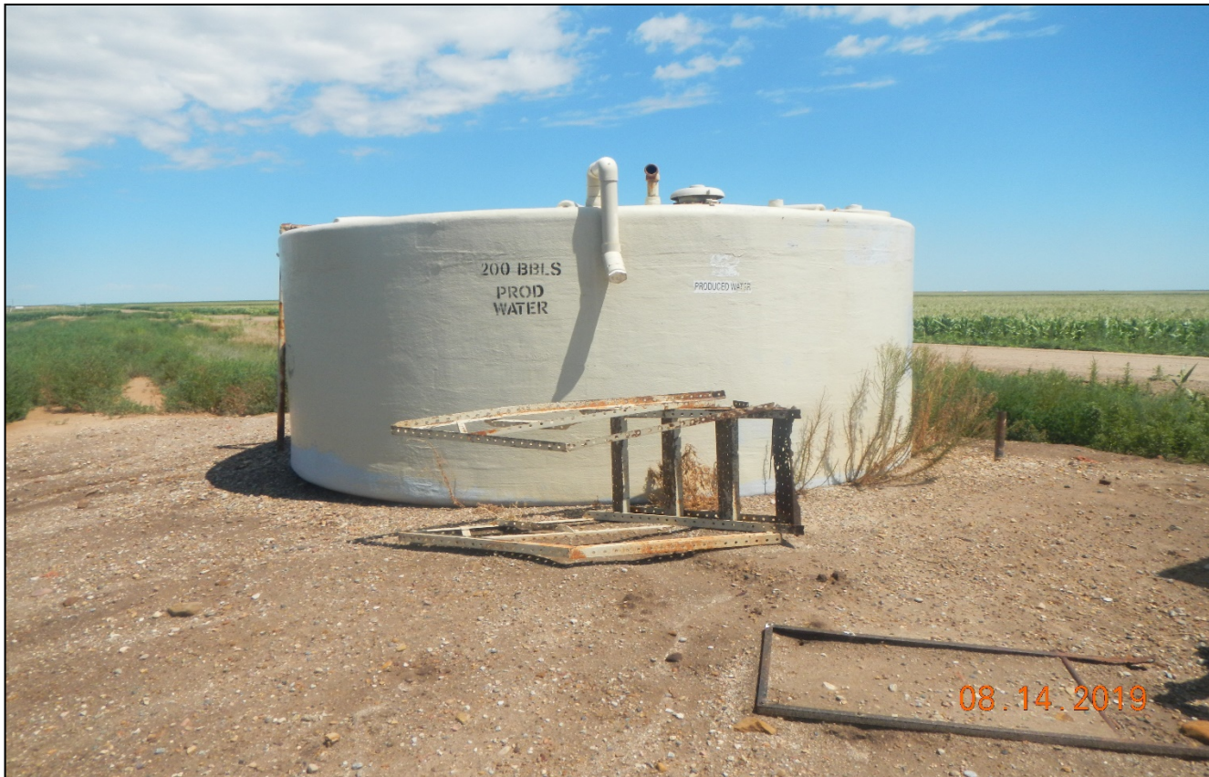
Photo 3. There is no berm around the 200 bbls tank. There is unused equipment at the location.
