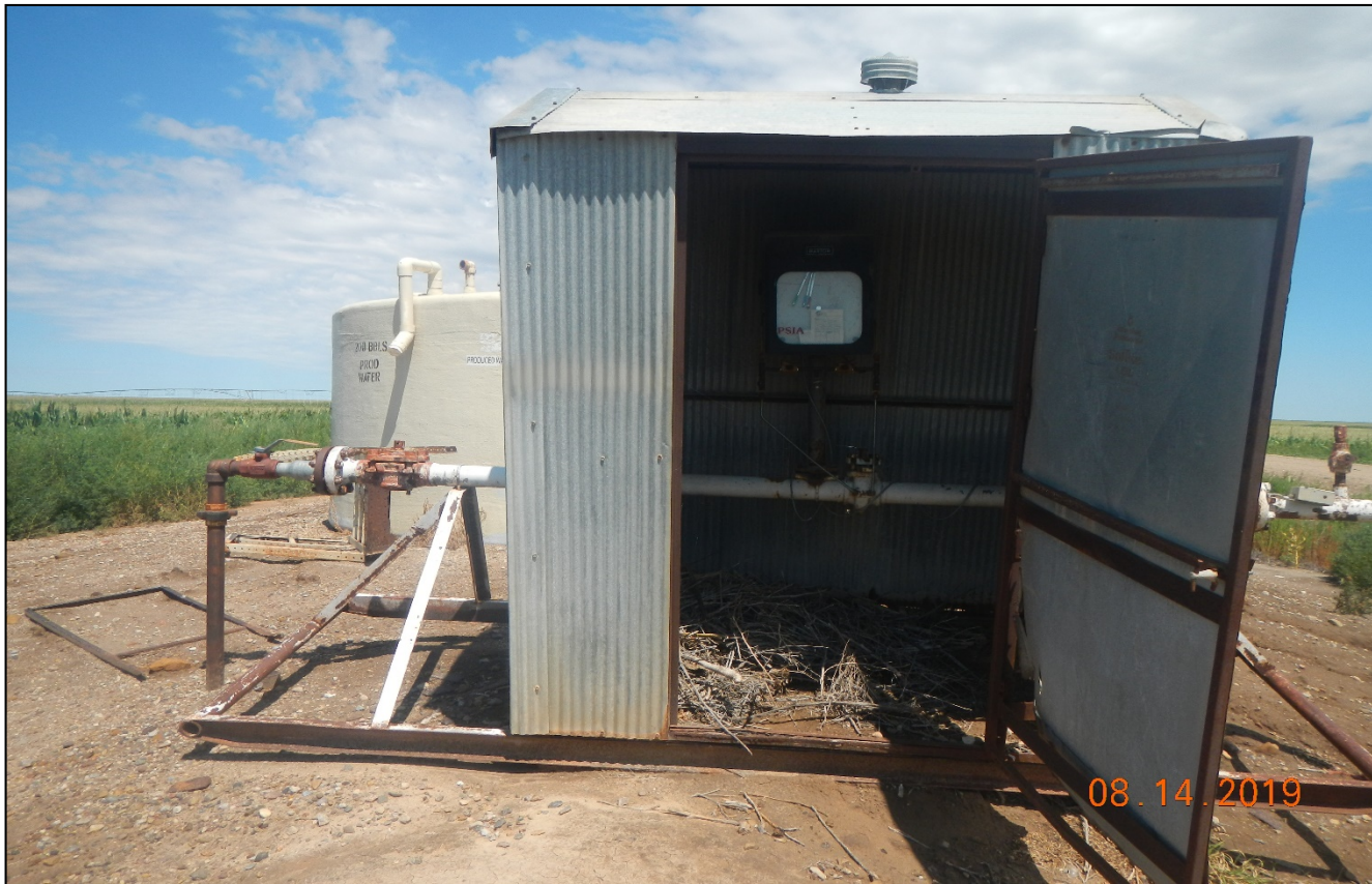
Photo 2. There was a hissing sound and strong odor around the meter shed. Operator was notified by phone the next day. The door is left open at shed and a lot of debris is inside.
