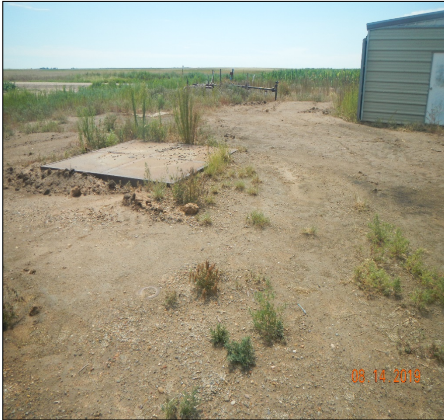
Photo 3 & 4. The pipe risers at the east side of the location were removed. Cement pads remain.
