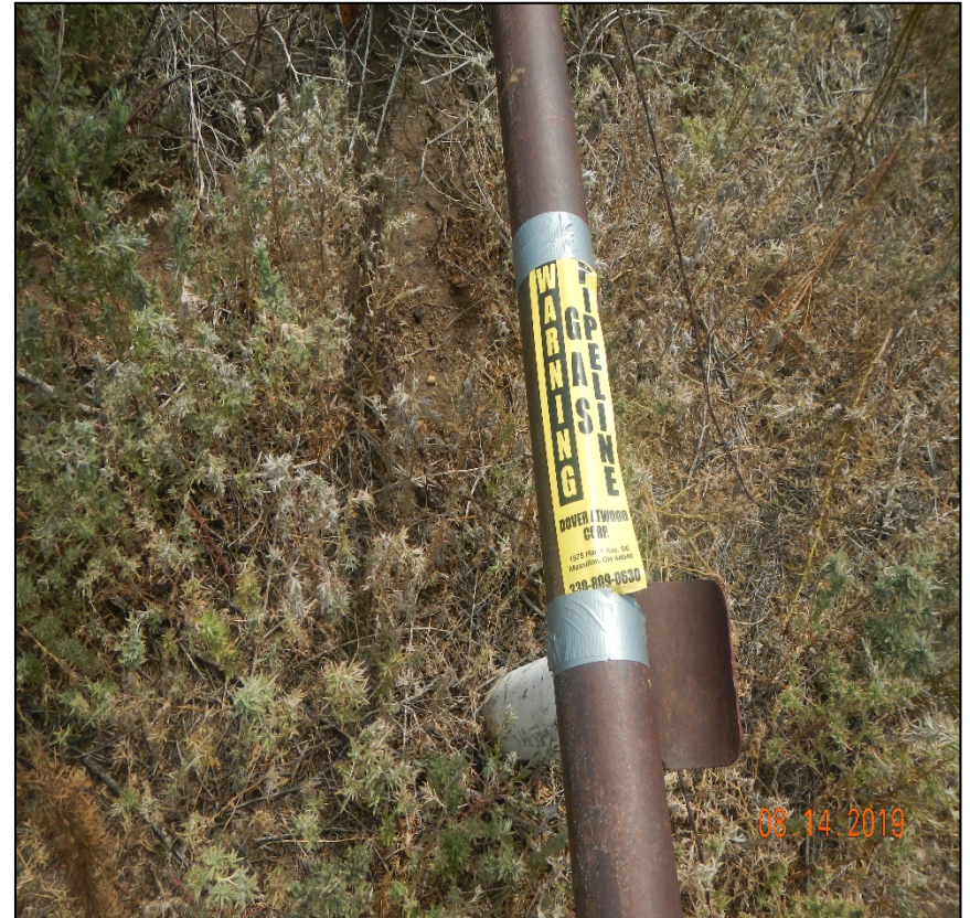
Photo 5 & 6. There is a gas pipeline that remains at the southeast corner of location. Operator sign is taped to the pipeline. This is not a permanent sign and is not sufficient.
