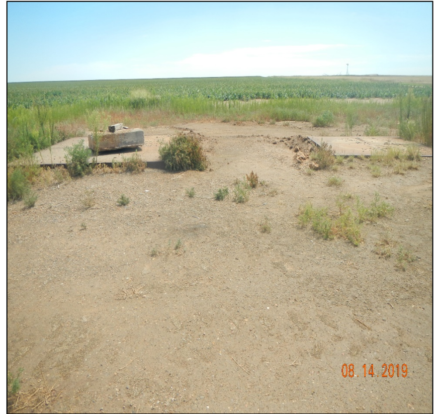
Photo 3 & 4. The pipe risers at the east side of the location were removed. Cement pads remain.
