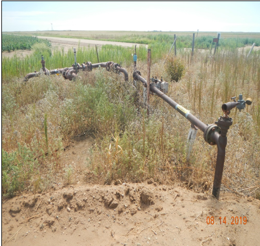
Photo 5 & 6. There is a gas pipeline that remains at the southeast corner of location. Operator sign is taped to the pipeline. This is not a permanent sign and is not sufficient.
