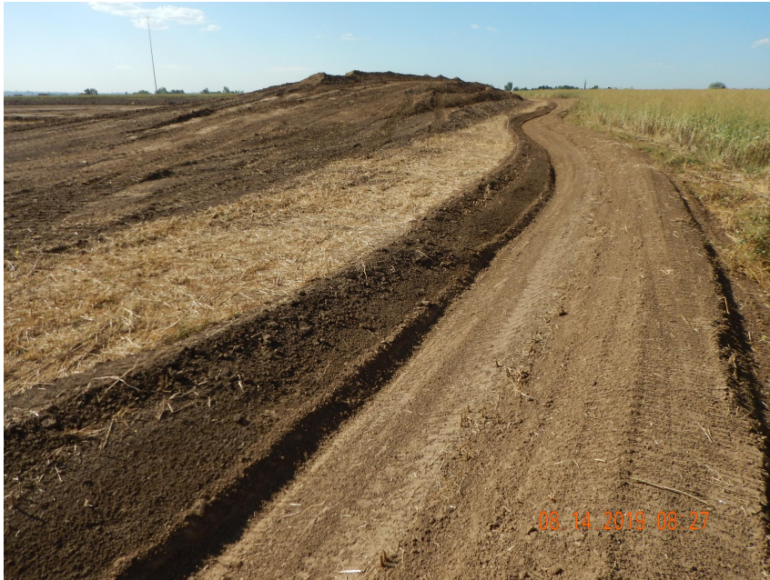
Photo 1. Photo taken from the northwestern location, facing South. Photo illustrates the perimeter ditch and berm BMP that has been installed around the entire perimeter of the location. At the time of this inspection, the perimeter BMP appears to be stabilized and in proper functioning condition during major construction activities (i.e., topsoil salvage operations).
