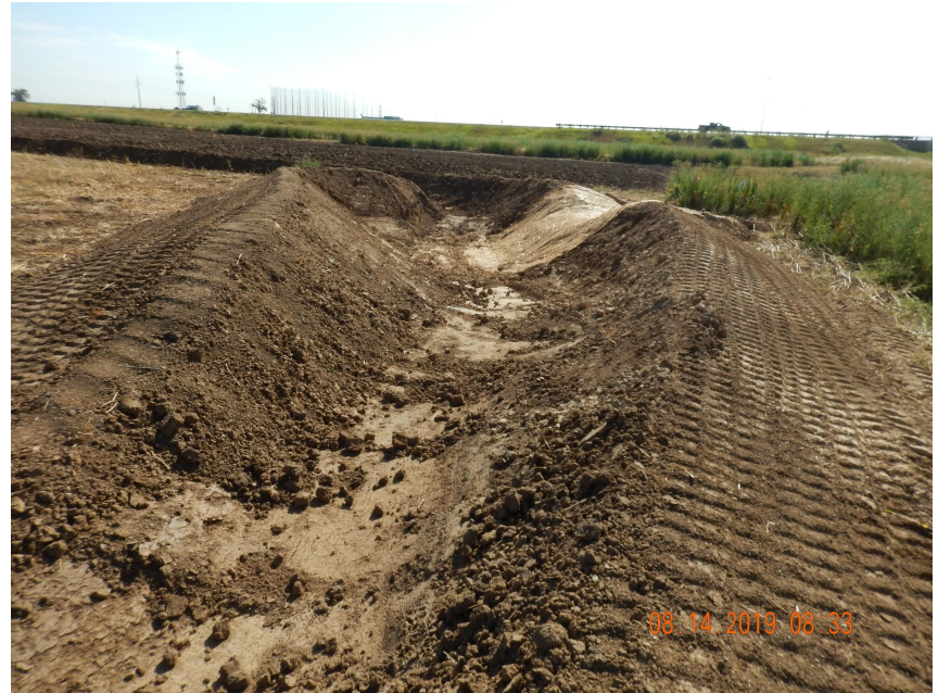
Photo 4. Photo taken from the southeastern location, facing East. Photo illustrates a sediment trap installed in conjunction with the perimeter ditch and berm BMP.
