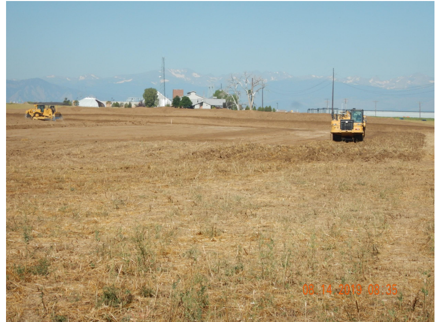
Photo 6. Photo taken from the eastern location, facing West. Photo illustrates topsoil salvage operations in-process.
