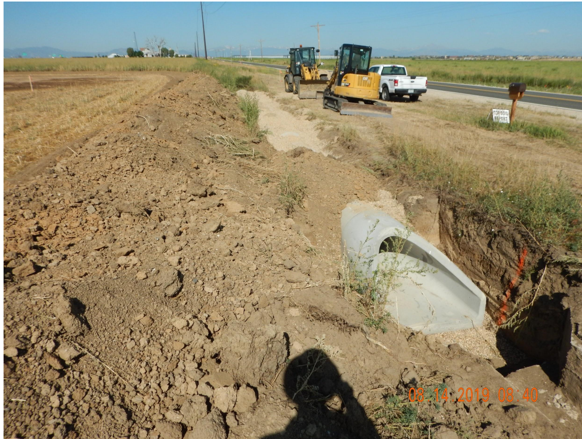
Photo 9. Photo taken from the northwestern location, facing West. Photo illustrates a culvert being installed along the roadside ditch for the access point to location.
