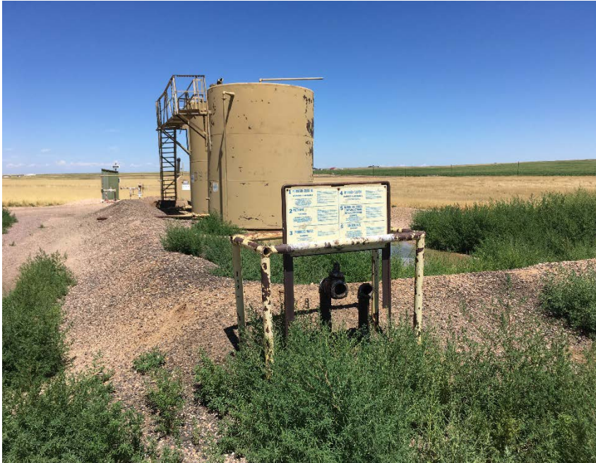
Tank Battery showing 1 – 300 BBL crude oil tank and 1 – 300 BBL produced water. Photo looking north. Very weedy.
