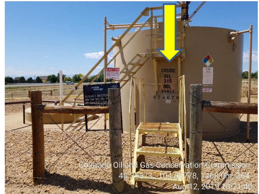
Photo 2: Tank Battery with labeling on tank
