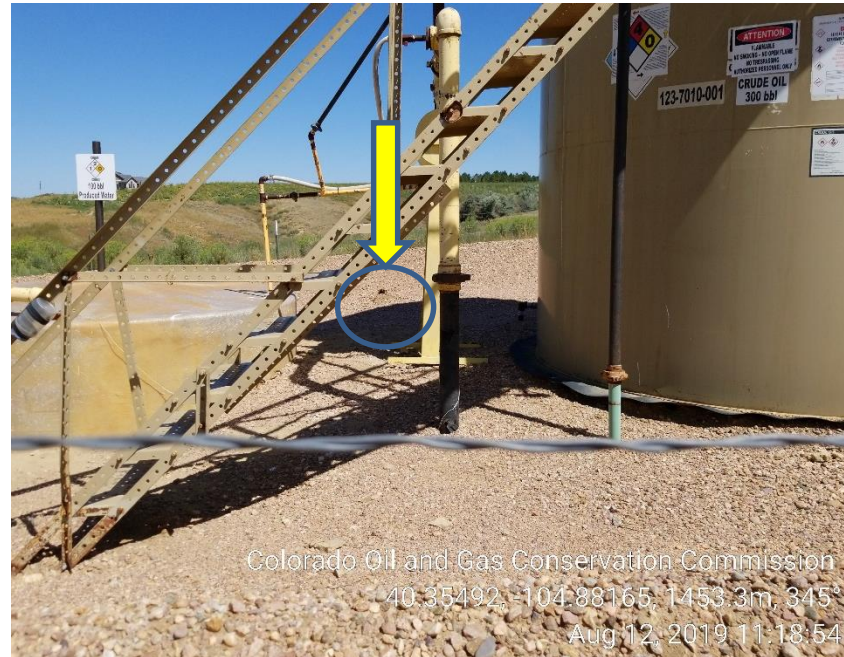
Photo 7: Hole in berm
