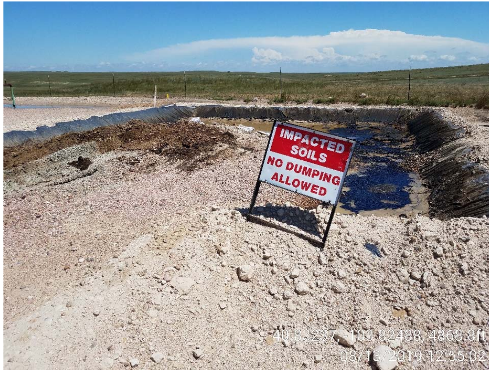
Photo 1 – Stockpile of impacted material from bermed lined containment. Free oil present.
