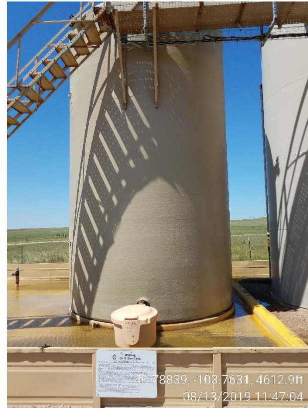
Photo 2 – Photo of new produced water AST, no placards or capacity/contents labeling present.
