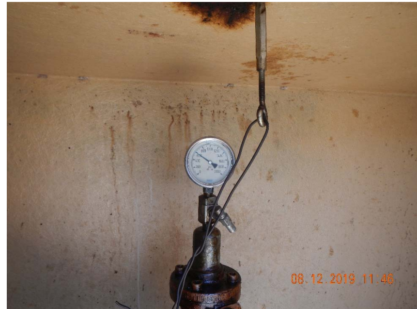
Photo 2. 600 psi on tubing at time of inspection.
