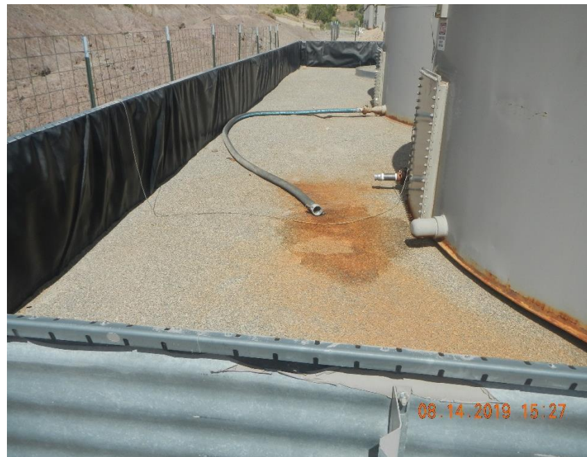
Stained gravel inside of tank battery containmnet.
