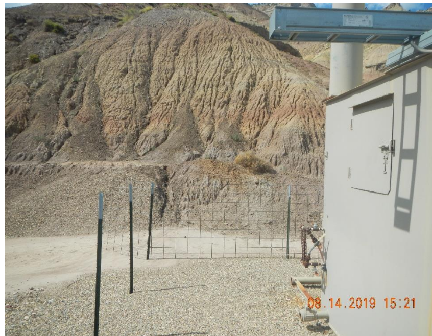
Sediment washing over diversion ditch behind separators.
