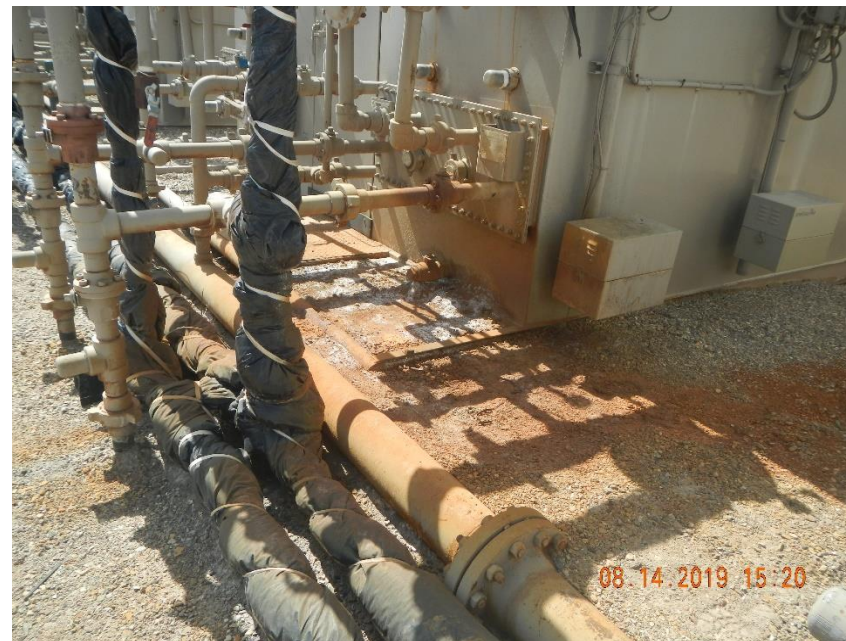
Stained ground surface at middle set of separators.
