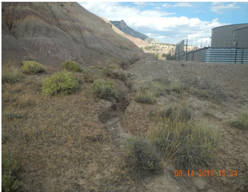
Diversion ditch from above tanks and battery flows out into field is washing and riling.
