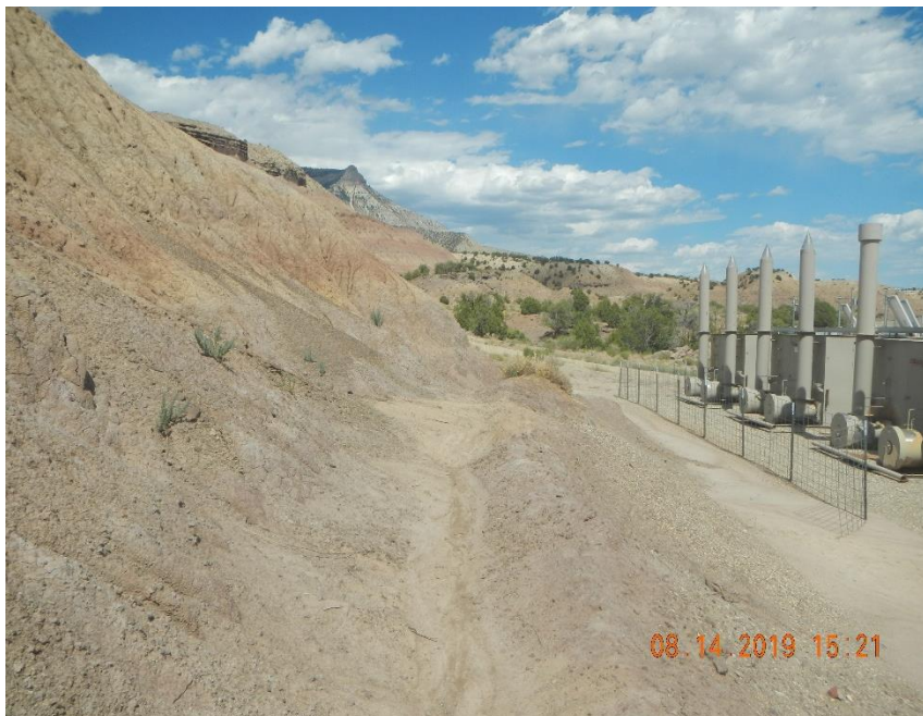
Sediment build up in diversion ditch behind separators and tank battery.
