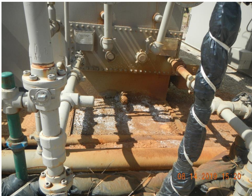
Stained ground surface at middle set of separators.
