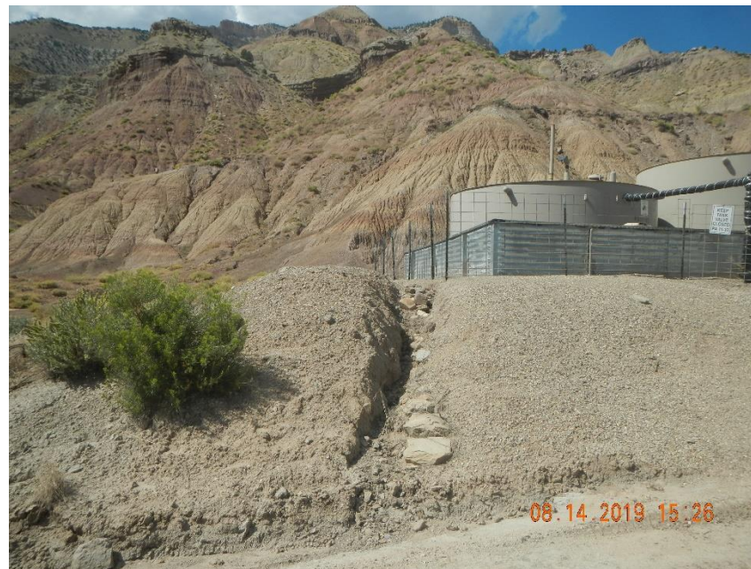
Diversion along tank battery is washed out.
