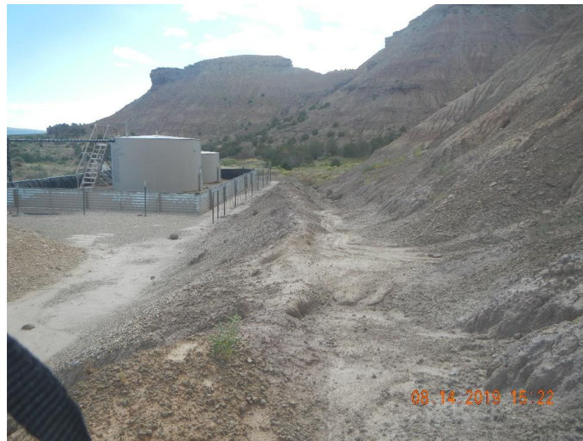
Sediment build up in diversion ditch behind separators and tank battery.
