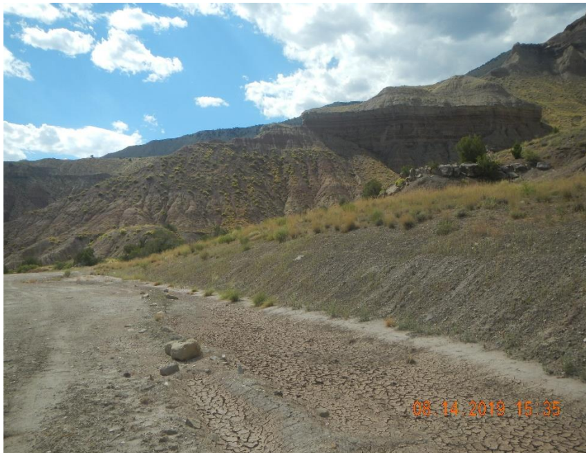
Cut slope on well pad not stabilized and washing sediment onto location.
